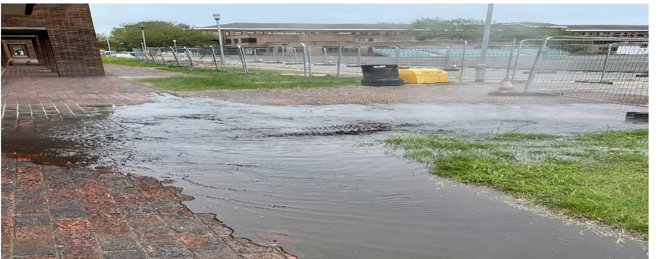
Photograph 3: Impacts of fluid leak on the local environment and drainage system
