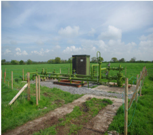
Existing brine wellhead at Holford Brinefield
