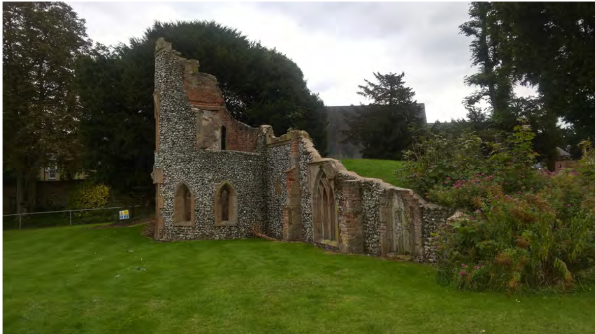
Picture 1.19 The Folly, Elm Grove - A Grade II listed structure which has benefitted from consolidation works and repairs.
