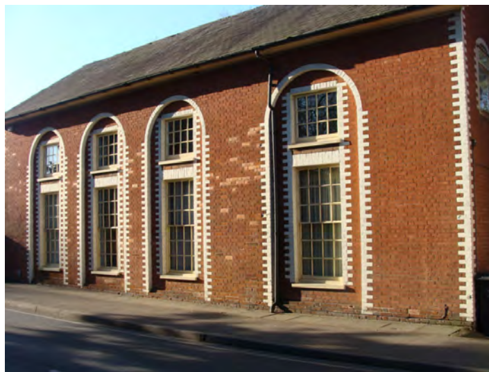
Picture 1.42 The Old Chapel, London Road; a listed building of distinction
