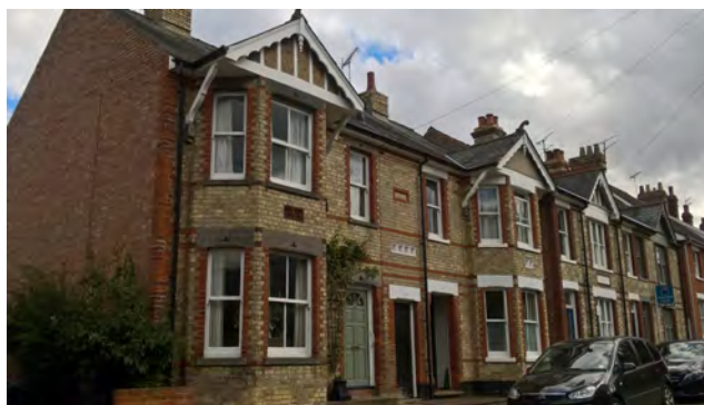
Picture 1.37 No.s 46 - 52 Fairycroft Road
