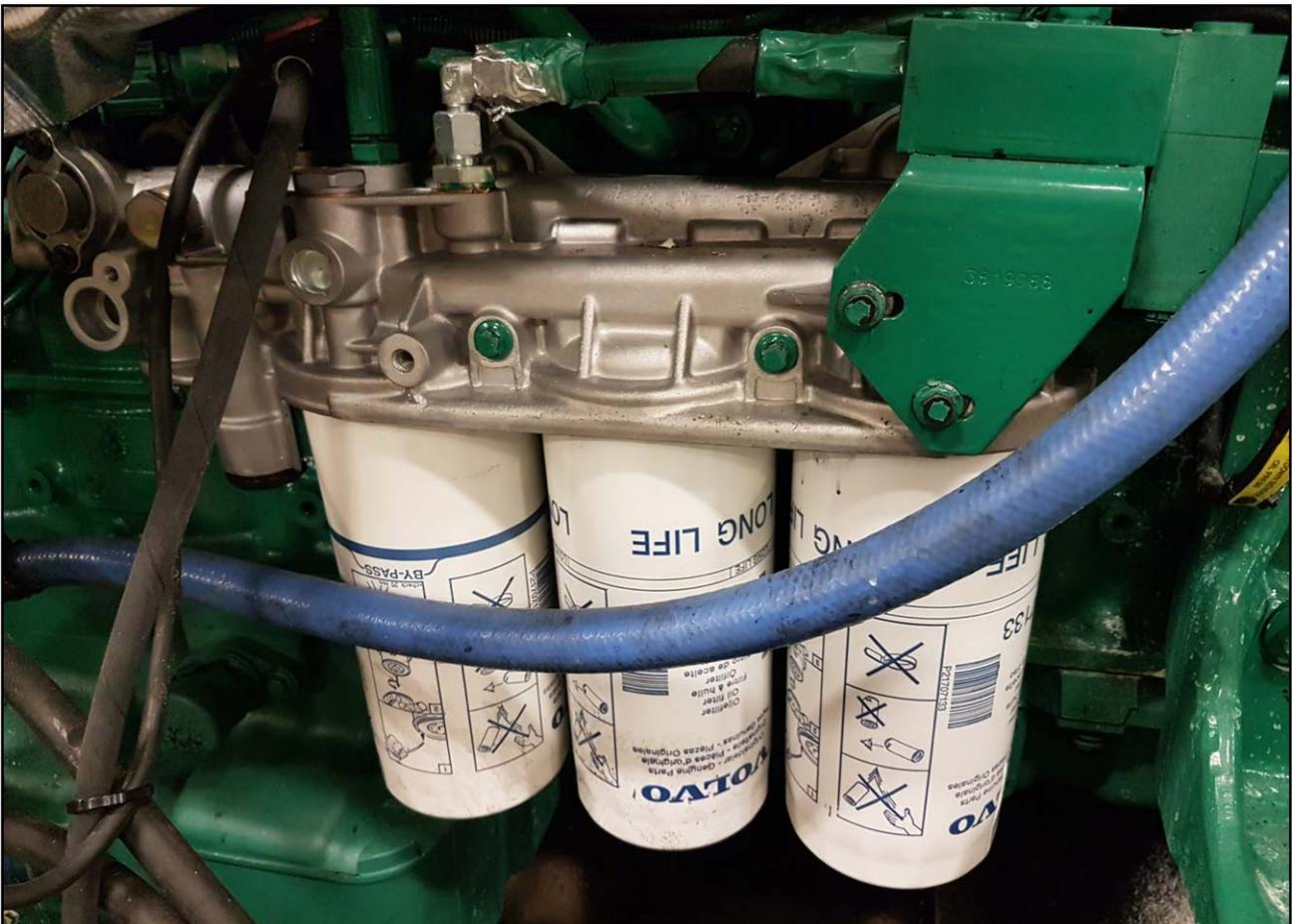
**Figure 20:** Replacement lubricating oil filters without changeover cock
