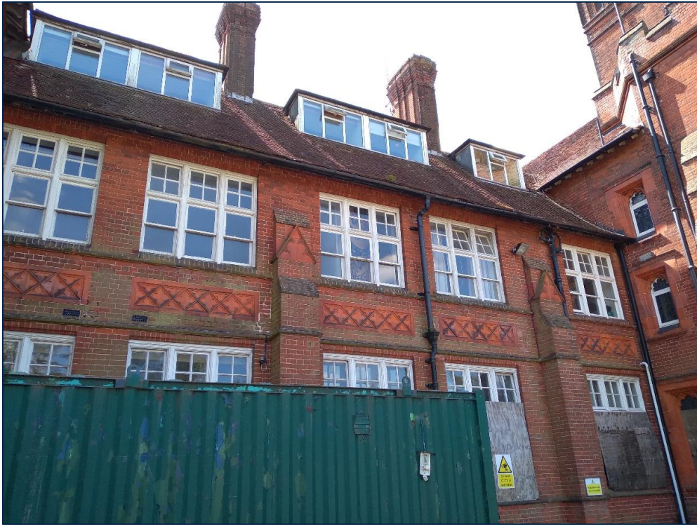
Figure 14: Photograph of east flanking wing, north elevation
