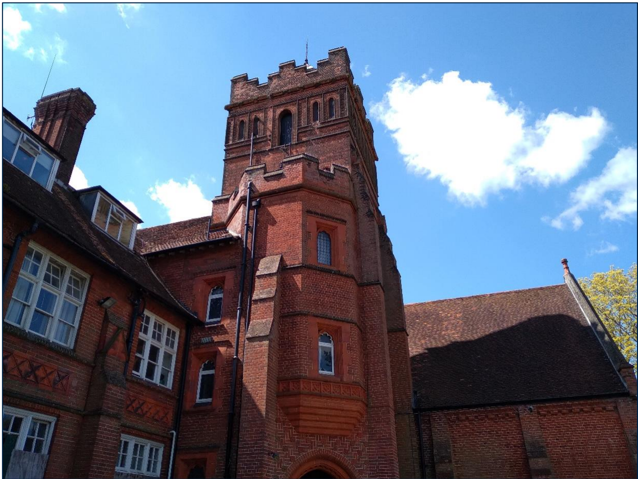
Figure 13: Photograph of central turret, north elevation
