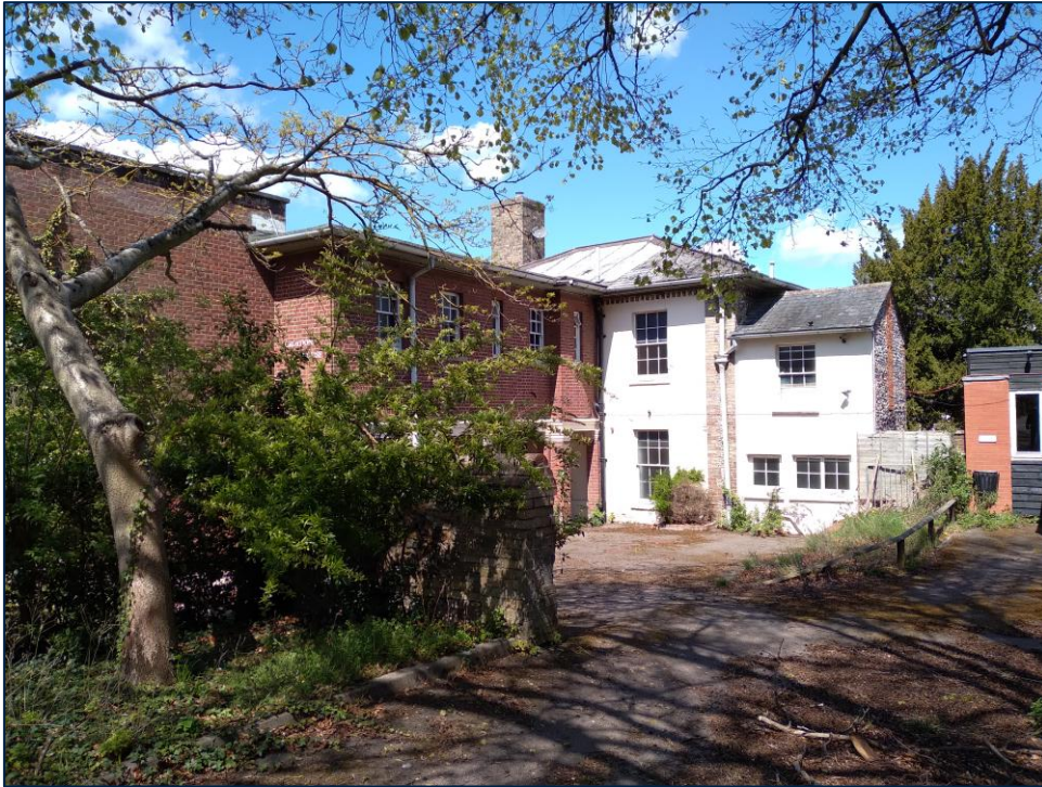
Figure 18: Photograph of Croydon Building
