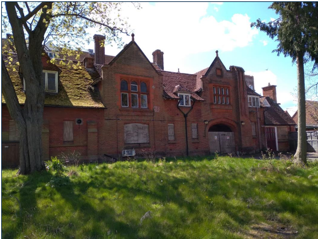
Figure 15: Photograph of west flanking wing, north elevation
