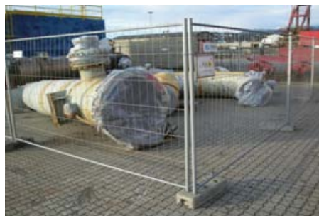
Figure 51. Material containing Asbestos which have been isolated before transport to final disposal site
