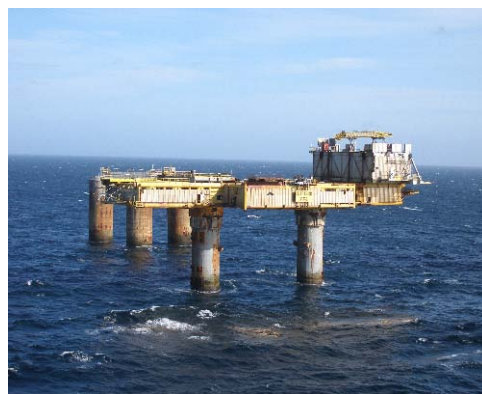
Figure 34. Last module ready for removal by S7000
