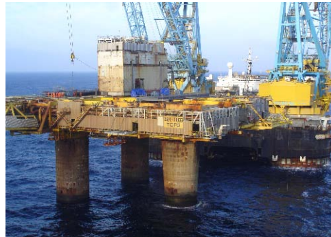
Figure 20. Last module being lifted off TCP2 MSF
