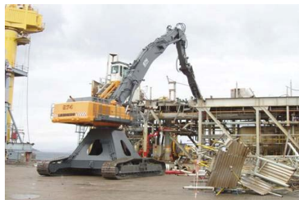
Figure 49. Demolition of modules using large excavators
