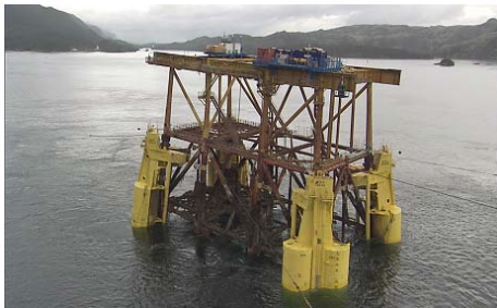
Figure 11. DP2 Jacket and MSF tow arriving the inshore location
