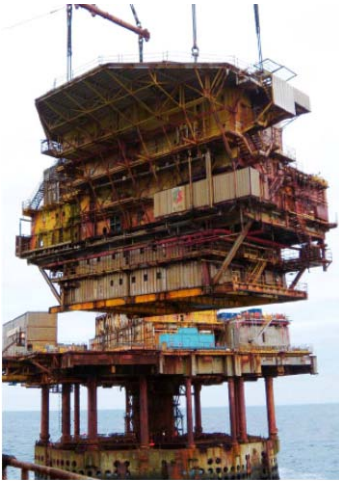
Figure 41. Four modules in one combine lift
