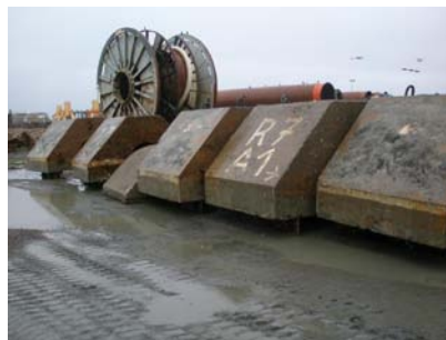
Figure 44. Concrete saddles removed from pipelines
