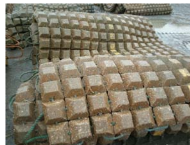
Figure 27. Concrete mattresses removed
