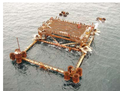
Figure 15. Work platform on DP1 jacket
