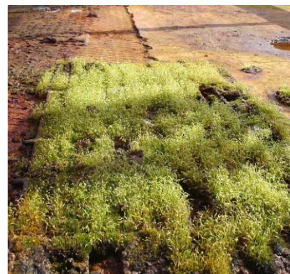
Figure 40. Grass found growing on the steel deck
