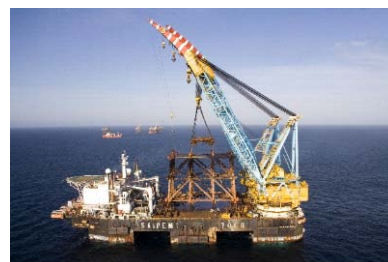
Figure 16. Upper part of DP1 jacket lifted off by S7000
