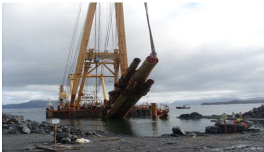
Figure 57. DP2 Jacket pile cluster (left) and QP jacket section (right) used as quay foundation at Aker Stord
