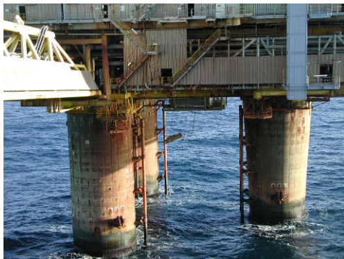
Figure 25. Before and after the removal of utility risers and ladders on one of the TCP2 concrete columns.
