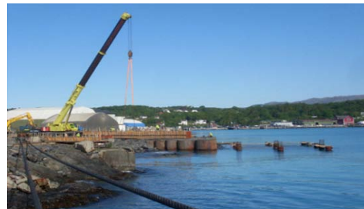
Figure 57. DP2 Jacket pile cluster (left) and QP jacket section (right) used as quay foundation at Aker Stord
