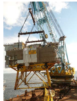
Figure 29. QP Topside and MSF being lifted onto the deck of S7000
