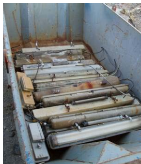
Figure 50. Sorted hazardous and EE waste material removed from modules for transport to waste handling contractor
