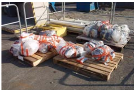
Figure 51. Material containing Asbestos which have been isolated before transport to final disposal site
