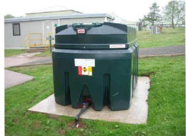
Integrally Bunded Plastic Above-ground Tanks
