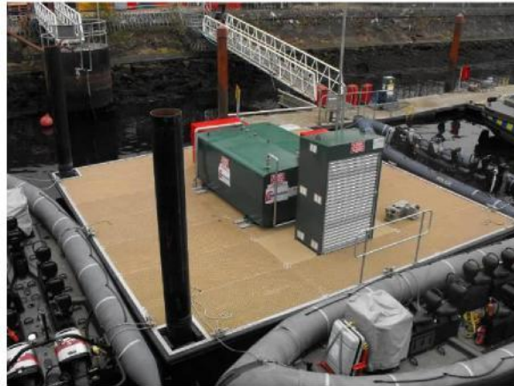
Typical Marine Refueling Installation
