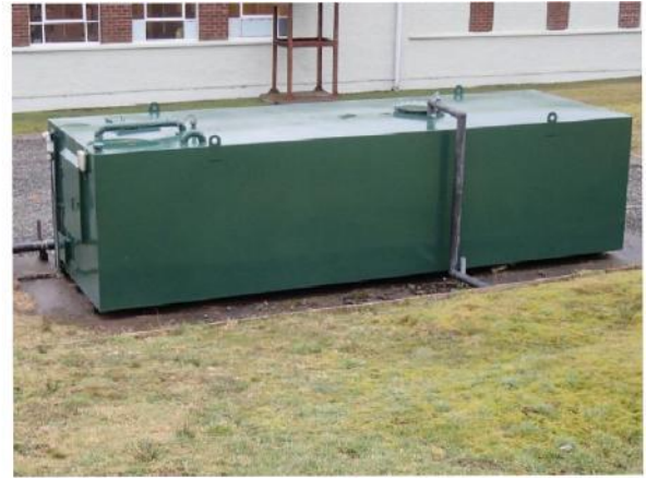
Above-ground Steel Single Skin Tanks
