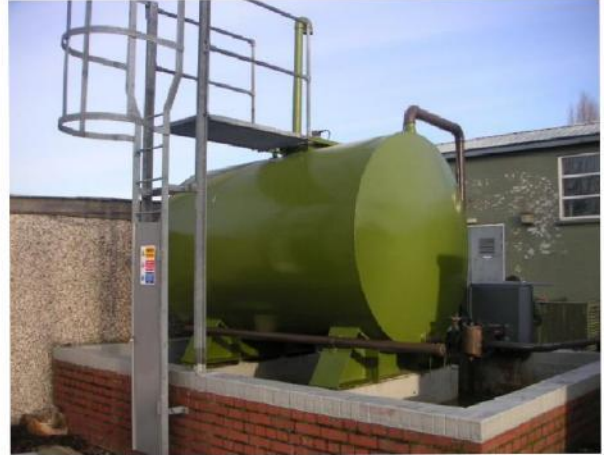
Above-ground Steel Single Skin Tanks
