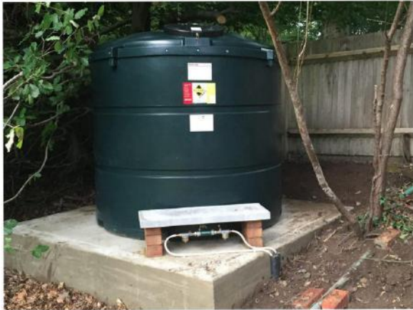
Integrally Bunded Plastic Above-ground Tanks
