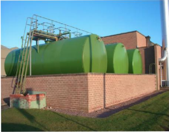
Above-ground Steel Single Skin Tanks
