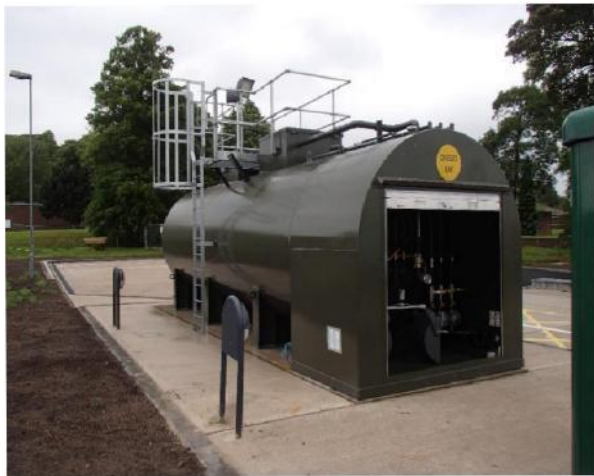
Integrally Bunded Steel Above-ground Tanks
