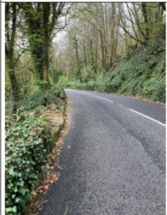
Figure 5: Example of lack of verge for step off.
