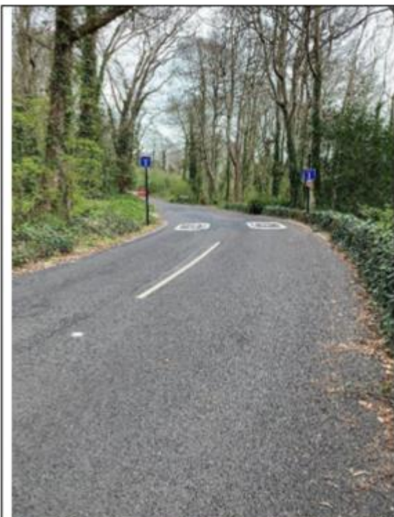
Figure 3: Close to location 2 looking eastwards to start of realignment of road.
