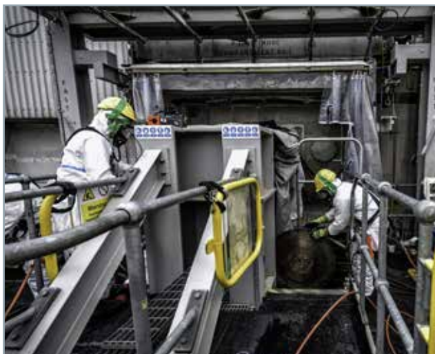
Doors being cut in the Pile Fuel Cladding Silo
