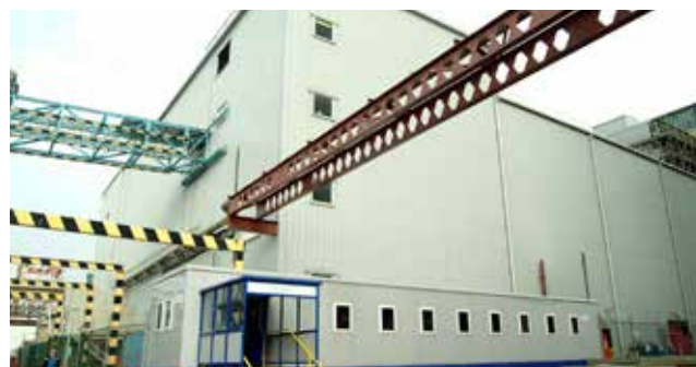
Magnox Reprocessing Plant - Sellafield End of reprocessing
