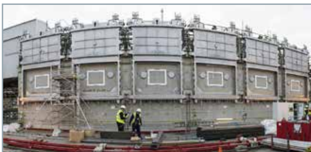
Pile Fuel Cladding Silo doors being installed
