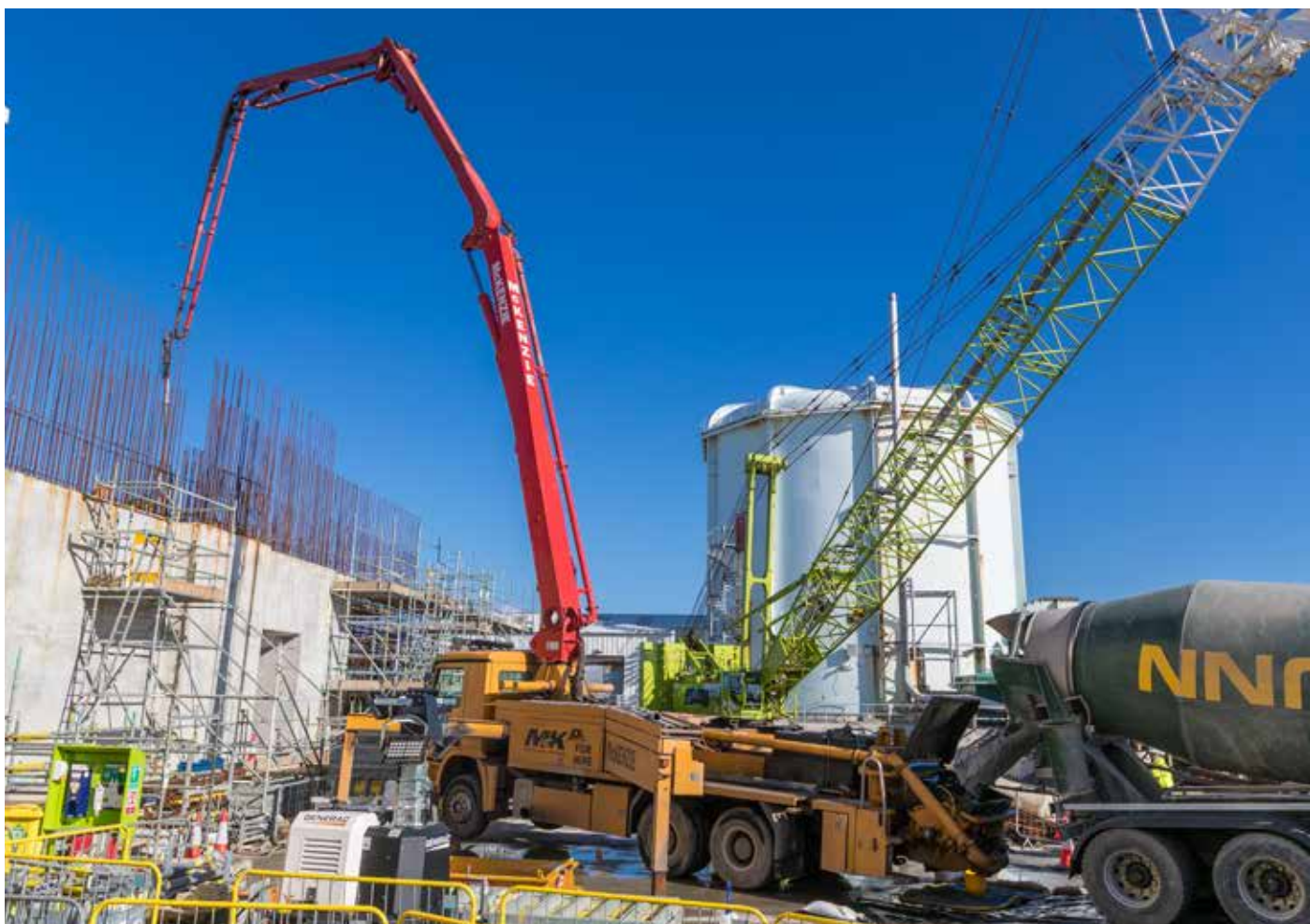
Work to construct the Doureay Cementation Plant store extension
