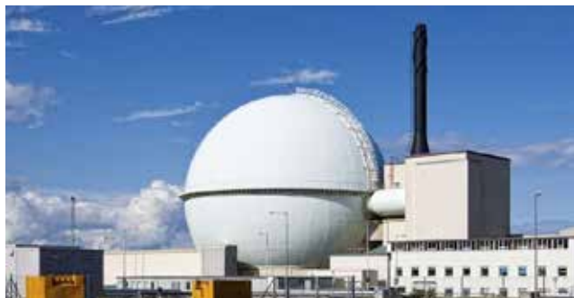
Dounreay Fast Reactor
