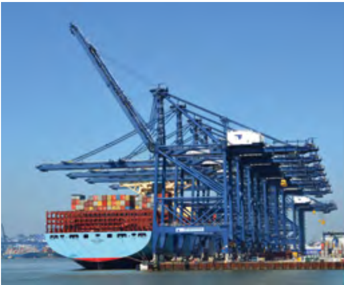
Large container ship being loaded at Felixstowe Port
