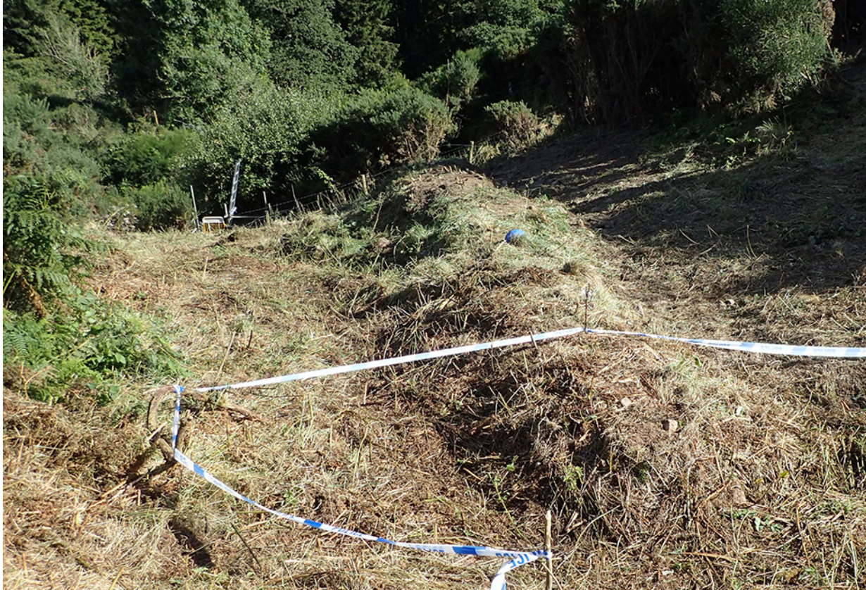
Figure 34: Bund viewed facing towards the 2011/12 drain post-accident after clearance of vegetation
