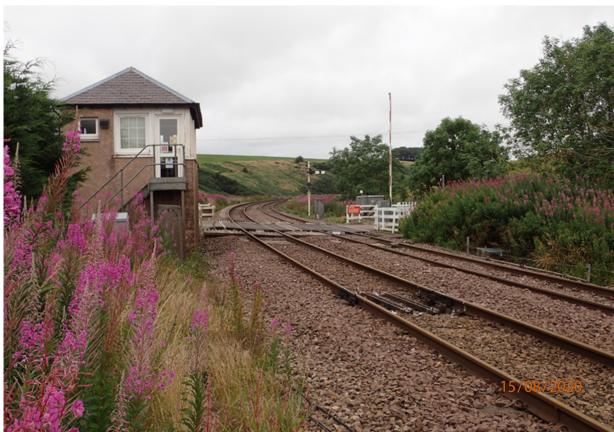
Figure 57: Carmont signal box looking north
