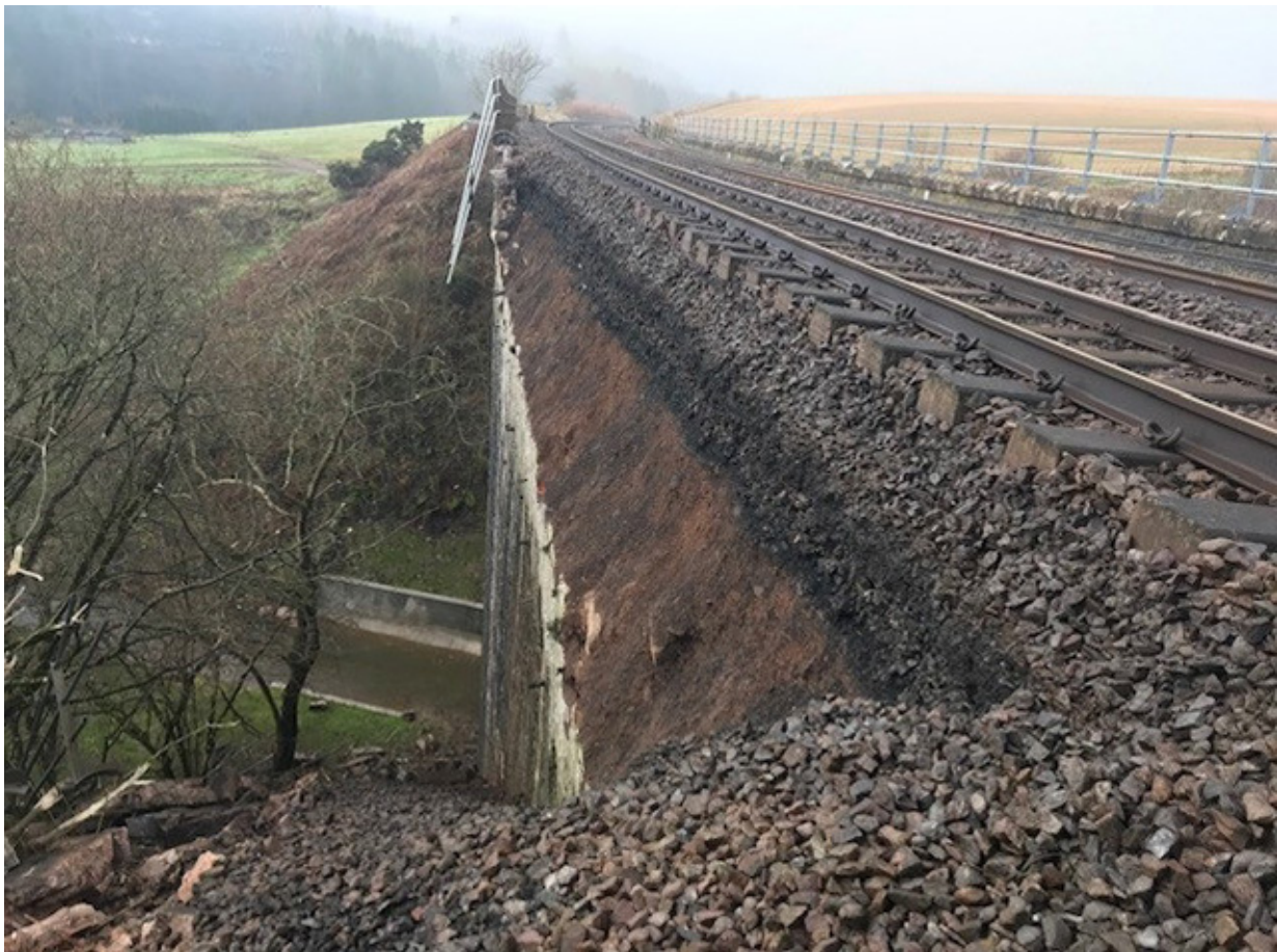
Figure M.2: Up line on bridge 328 looking south on 15 January 2021 (Network Rail)
