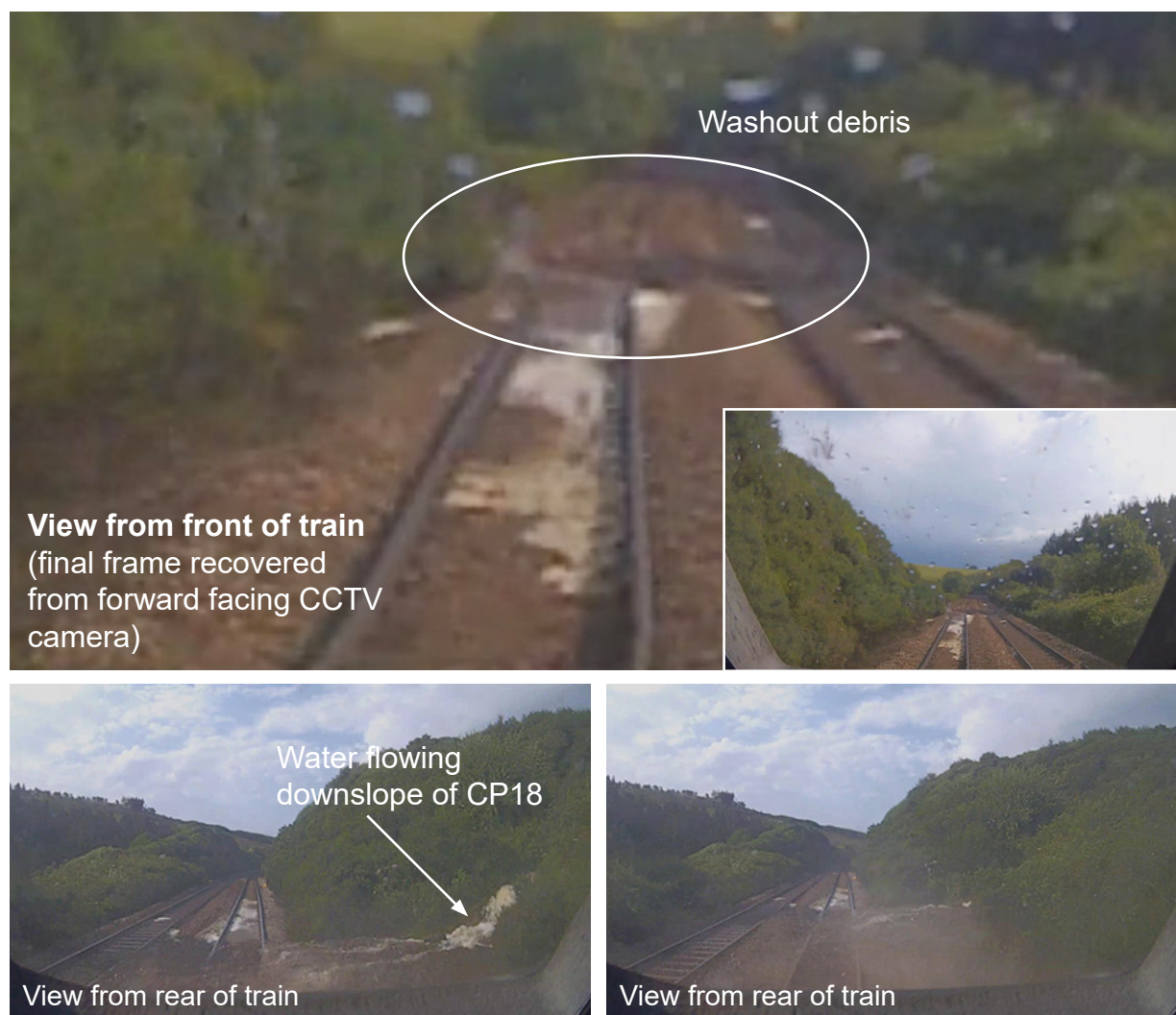
Figure 21: CCTV images from train 1T08 showing the washout (ScotRail)
