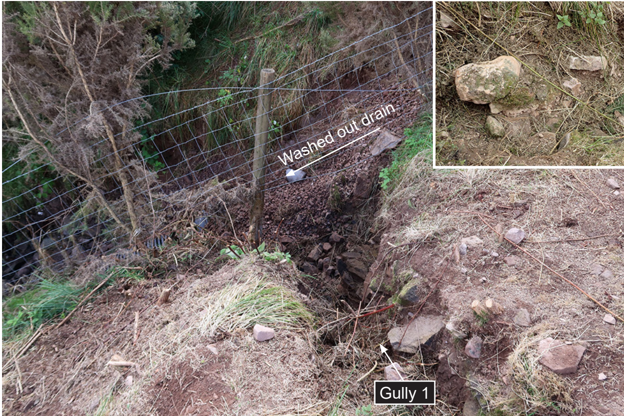
Figure 38: Gully 1 erosion at junction with 2011/12 drain (ORR/Coffey). Inset shows organic growth in base of gully 1 just outside main picture
