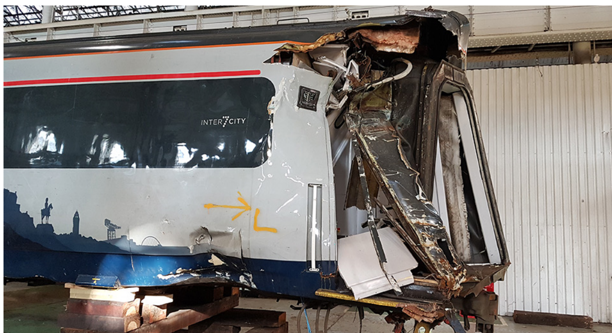
Figure 79: Damage to leading end of coach A
