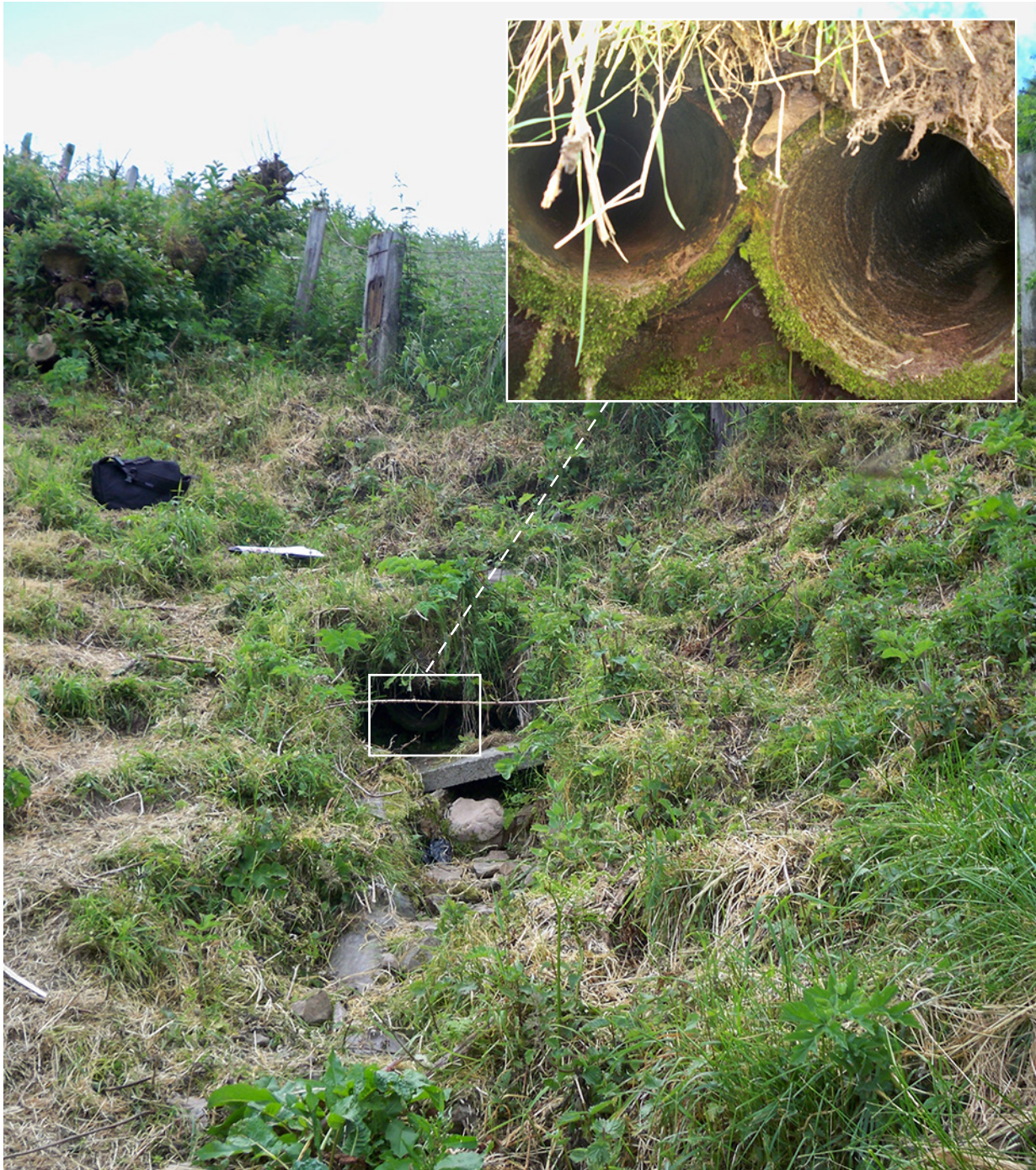
Figure 48: Pipes entering channel in pre-2010 drainage system at as-designed position of CP18 (Arup, June 2010). Inferred that left-hand pipe is from historic crest drain and right-hand pipe from pre-2010 drainage ditch as shown on figure 32
