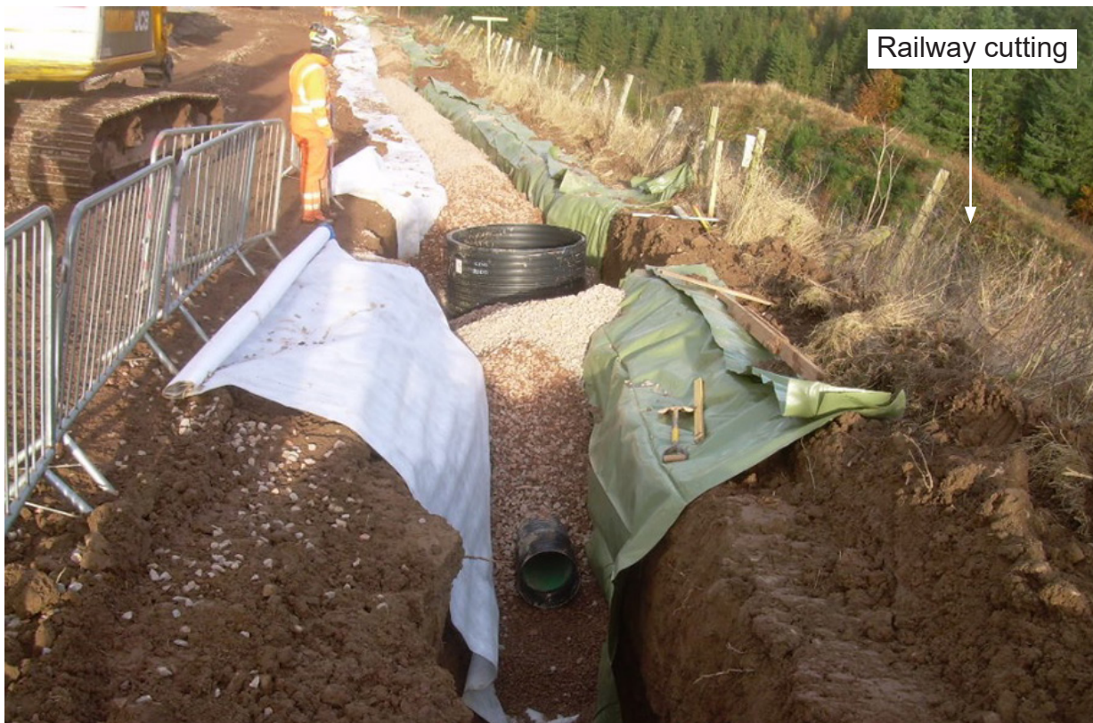
Figure 50: Drain under construction in late 2012 showing section between CP11 and CP16 looking north (Network Rail)
