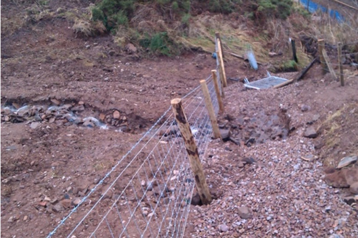
Figure 52: Surface of drain looking towards CP18 and railway in December 2012, before completion of the fencing (landowner)
