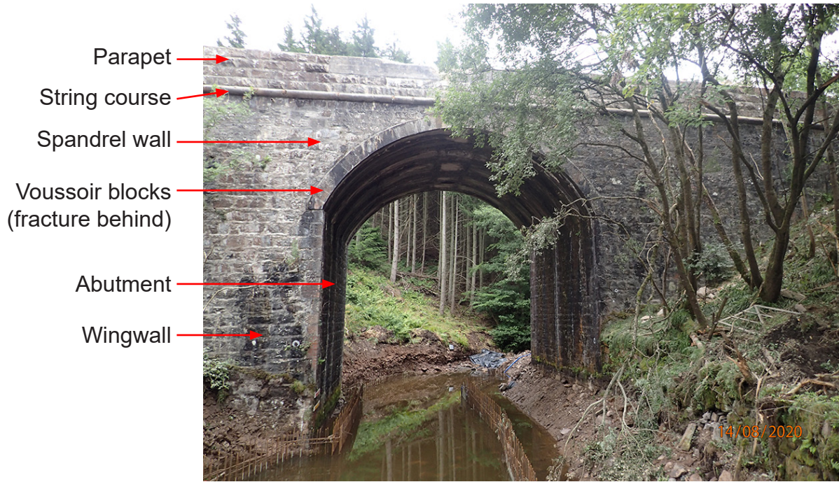
Figure F.7: Down-side elevation of bridge 325 on 14 August 2020
