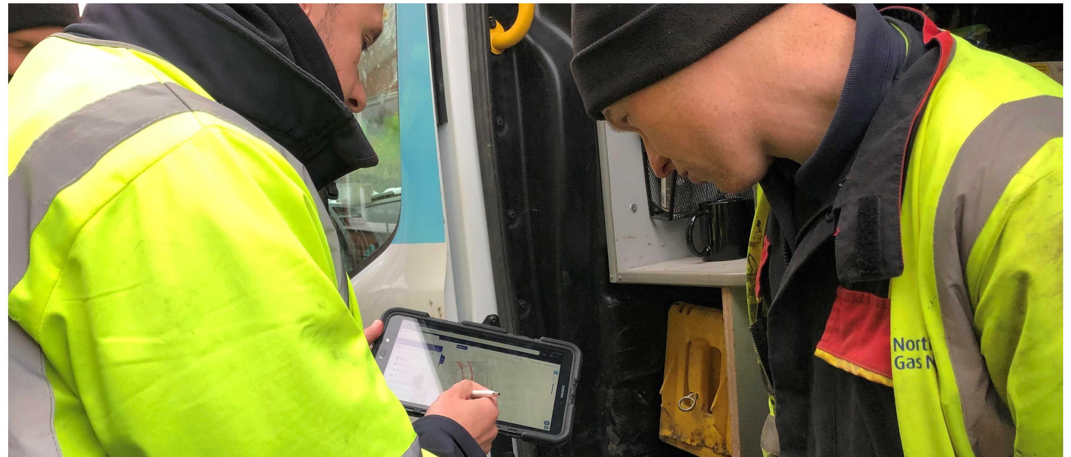
Engineers from Northern Gas Networks during field testing in the North East
