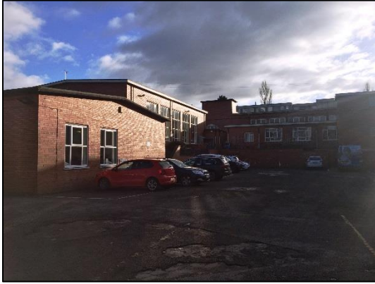
Existing buildings on site which will be demolished.
