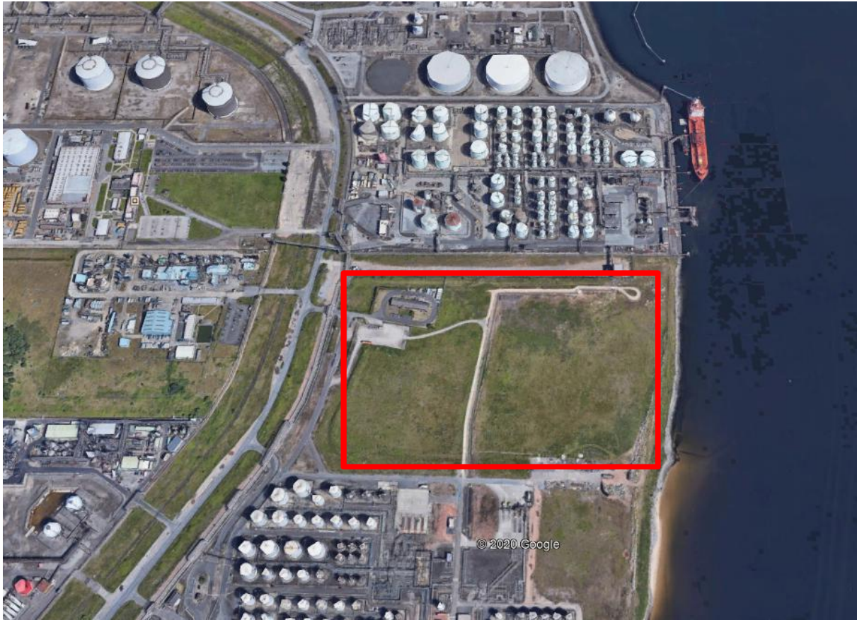
Figure 2-2 - Google Earth view of Potential Location for New CO 2 Marine Export Facility
