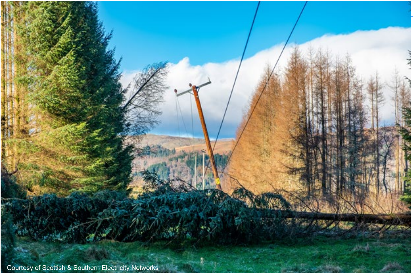
Photo 1: Overhead line damaged by fallen trees during Storm Arwen
