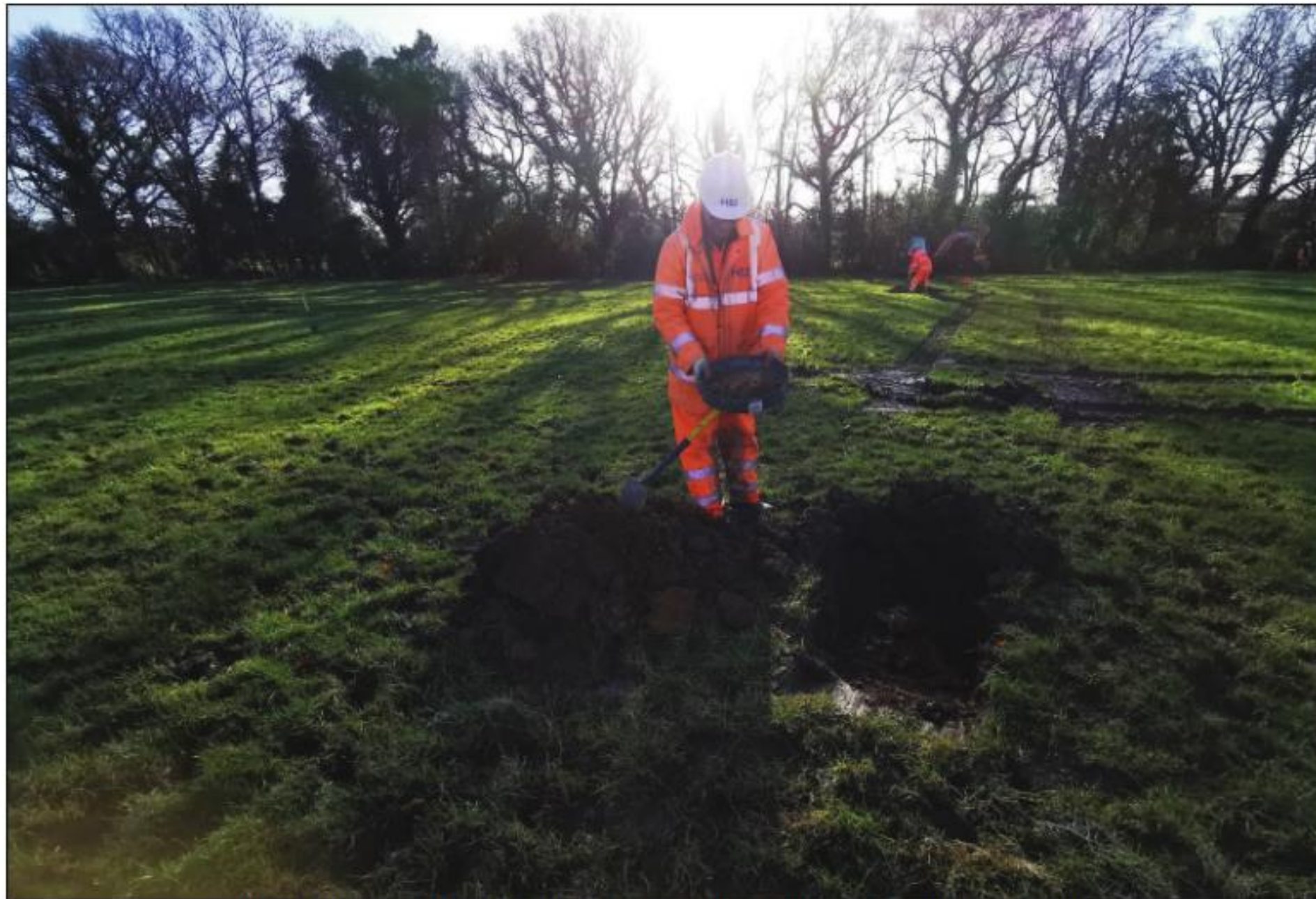
Plate 1 - Land Parcel C21044, Field 39 working shot, looking east.
