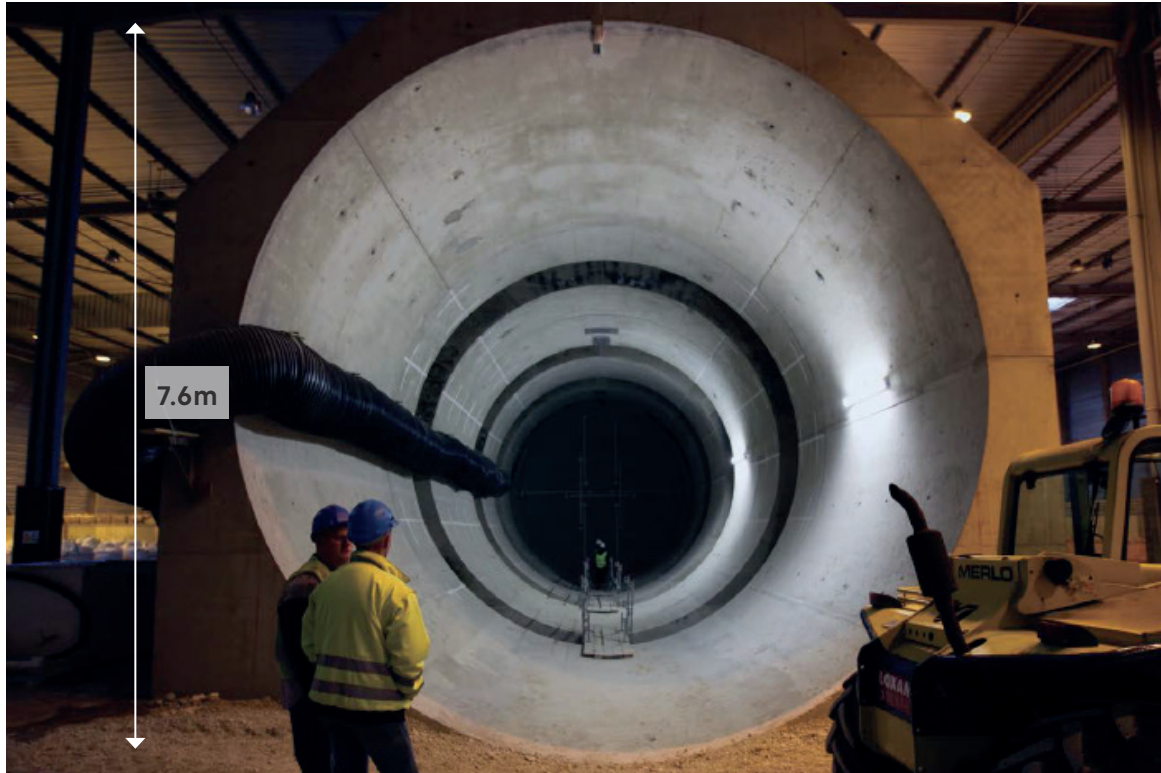
Figure 5: A full-scale seal experiment, part way through construction. Copyright Andra.
