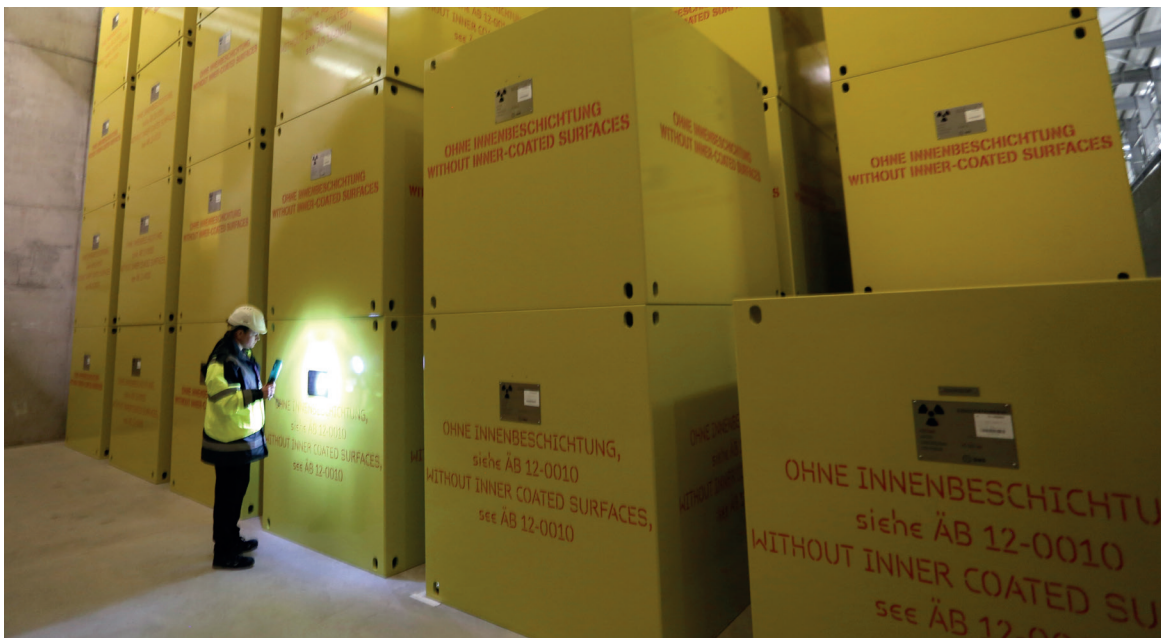
Figure 3: Intermediate Level Waste store at Berkeley.
