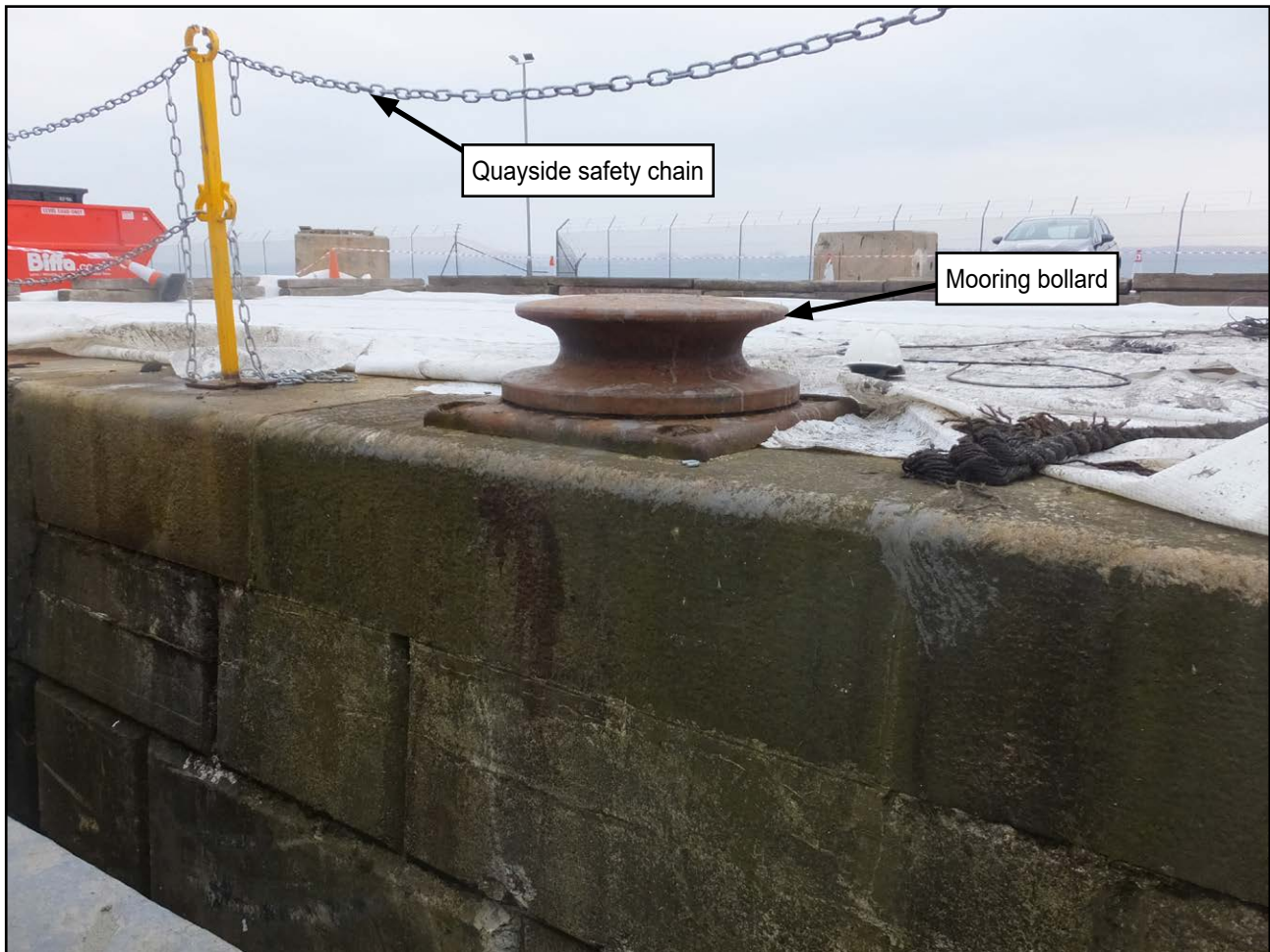
Figure 6: Quayside where the master was attempting to step ashore
