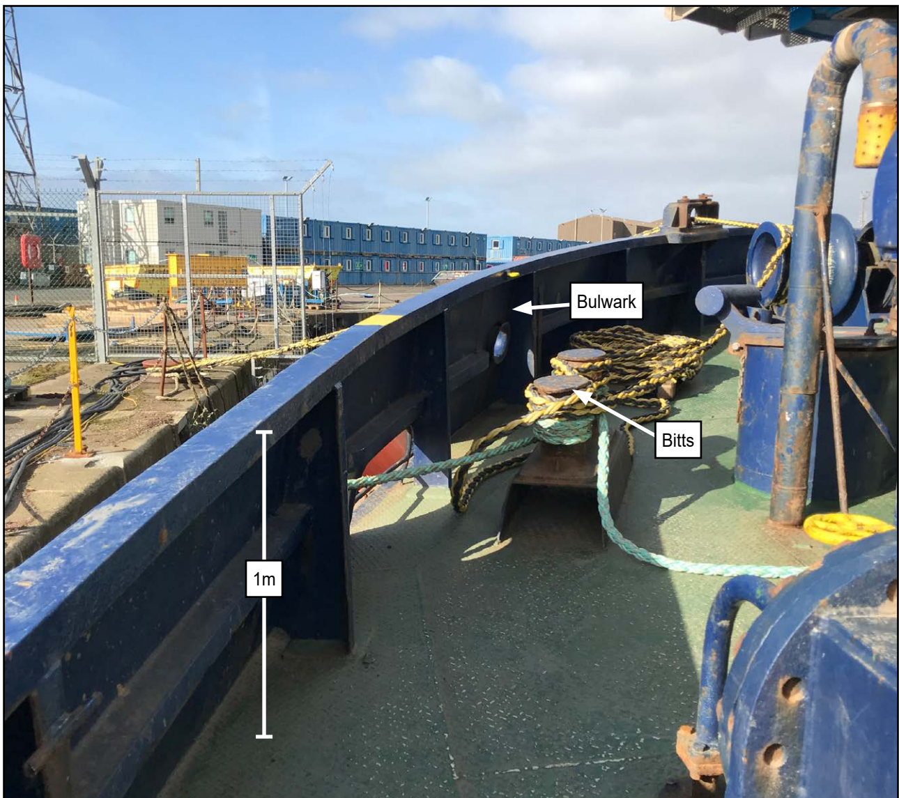
Figure 4: Cherry Sand fore deck bulwark and mooring bitts
