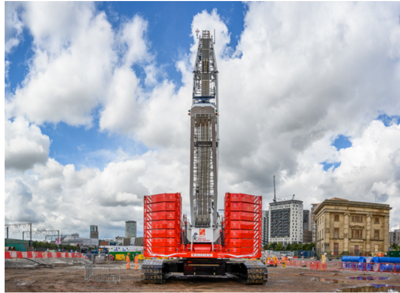
An electric crane at our site at Curzon Street, Birmingham.
