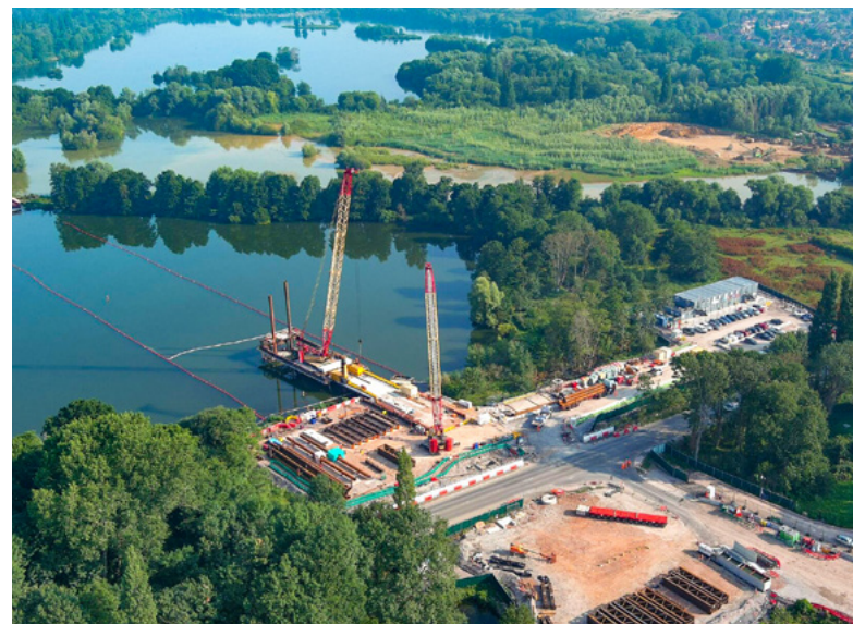
Drone footage of Colne Valley Viaduct jetty construction.
