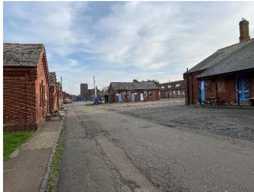
View through central part of the Site looking east
