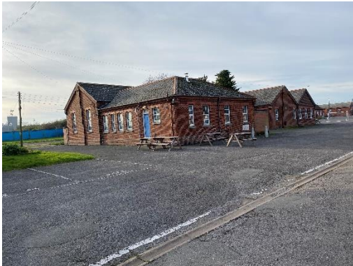
Typical single storey red brick buildings found on Site
