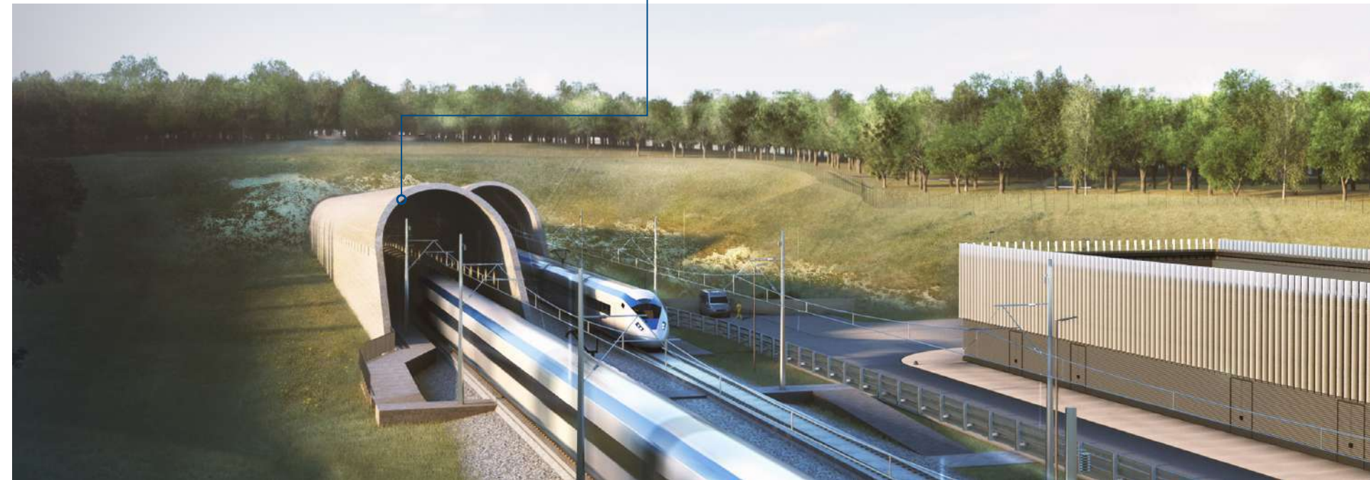
Curved architectural language of Chiltern Tunnel south portals integrated into the form of weathering steel viewing areas
