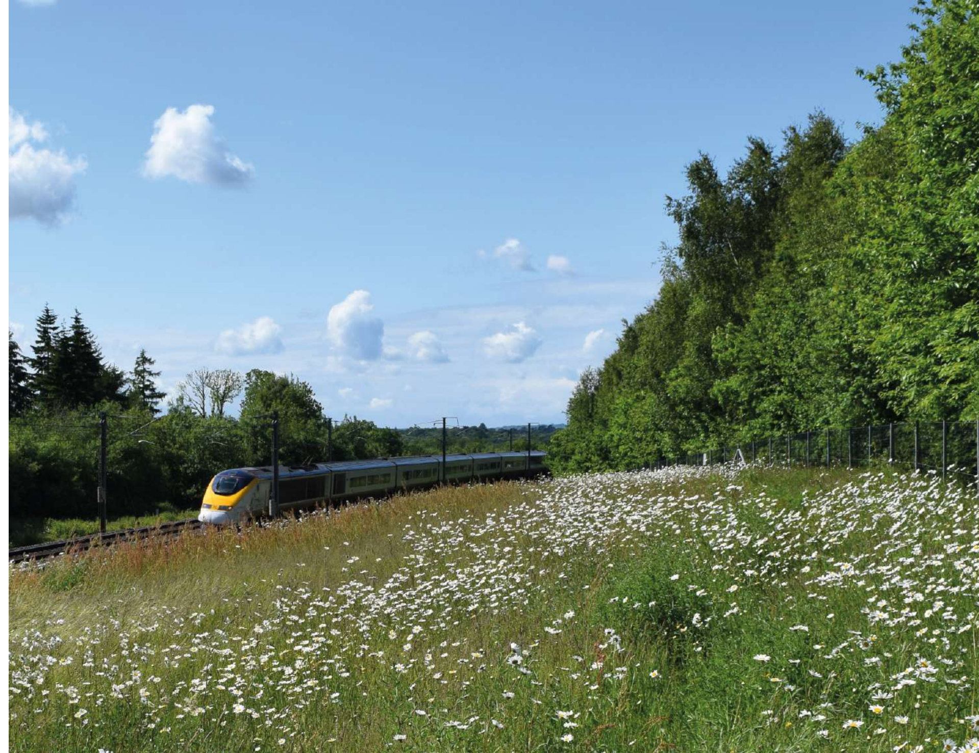
Fig.3.7_ Photograph - HS1 completed works (Arup)
