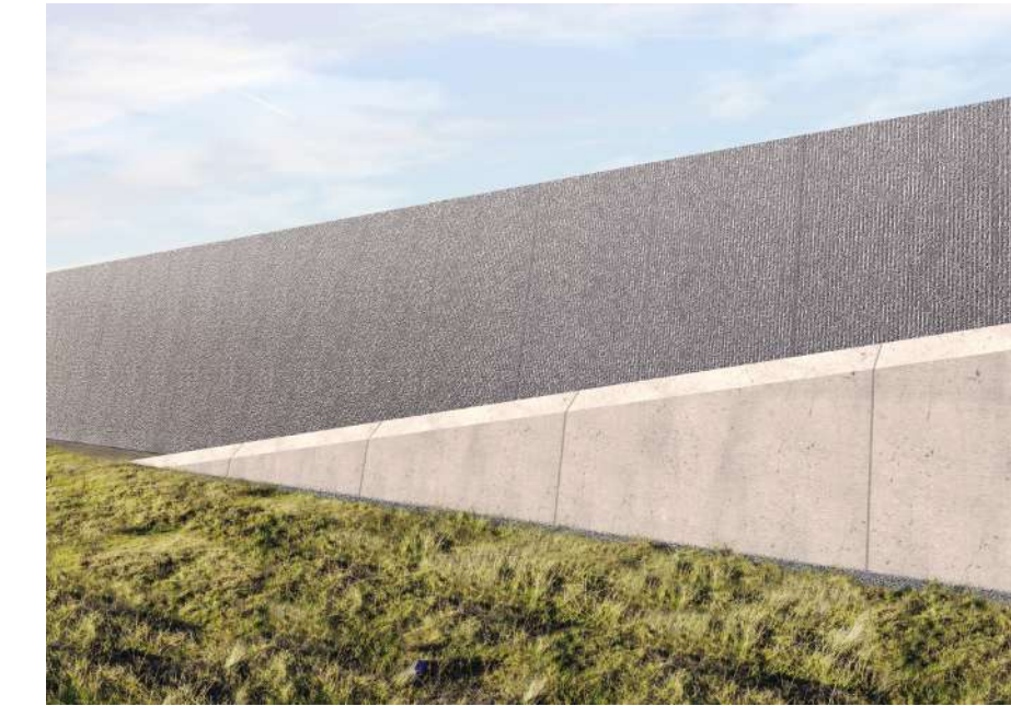
Fig.6.50_ Visualisation - View of embankment noise barrier detail
