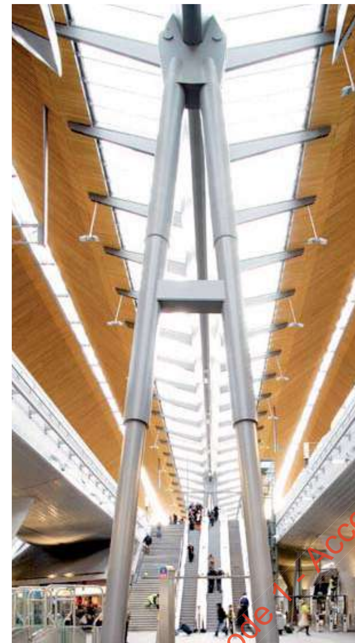
Fig.5.35 Oregon Pine soffits, Amsterdam Bijlmer ArenA station
