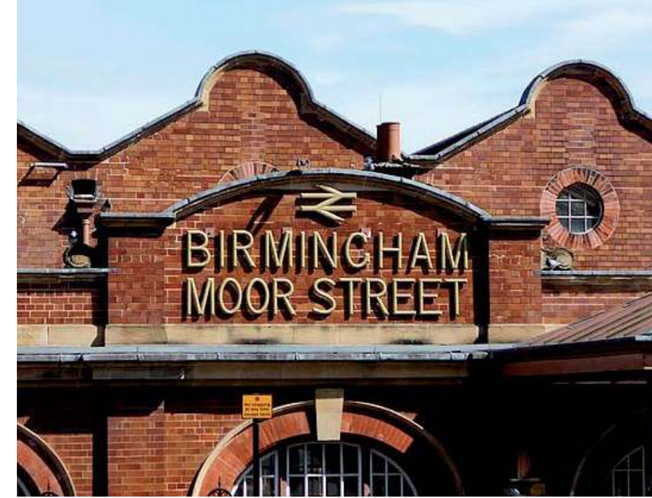
Fig.2.12 Birmingham Moor Street Station
