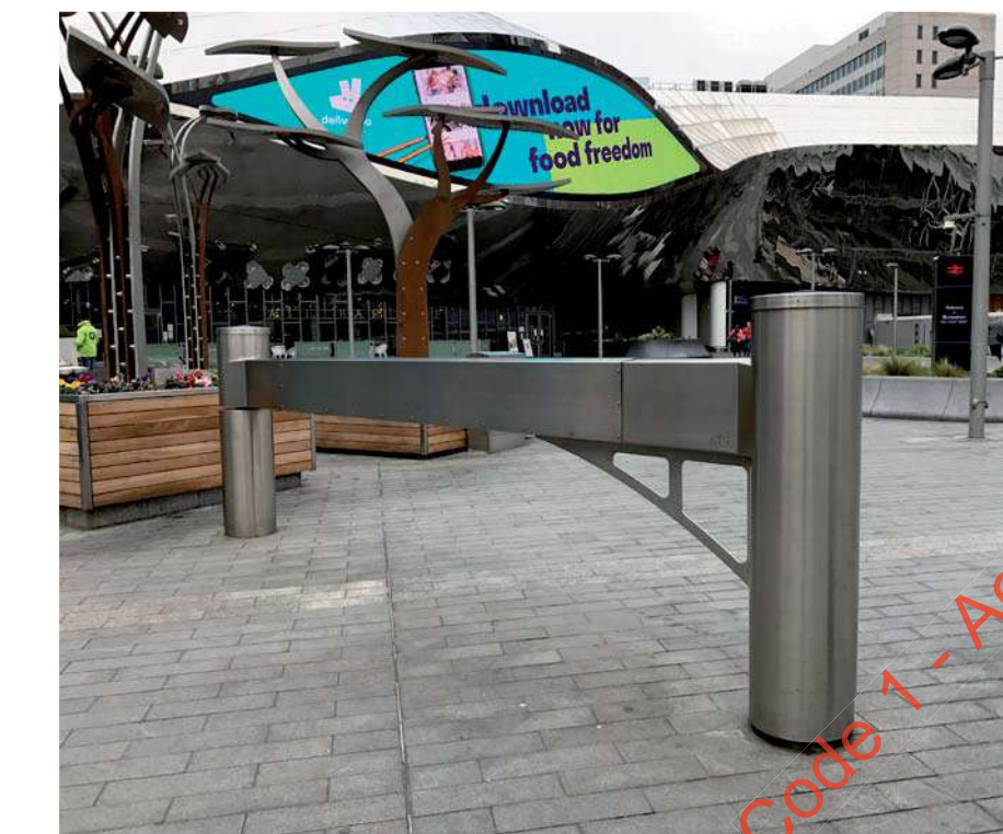
Fig.4.60 Example of operable features that can be coordinated with below ground utilities
