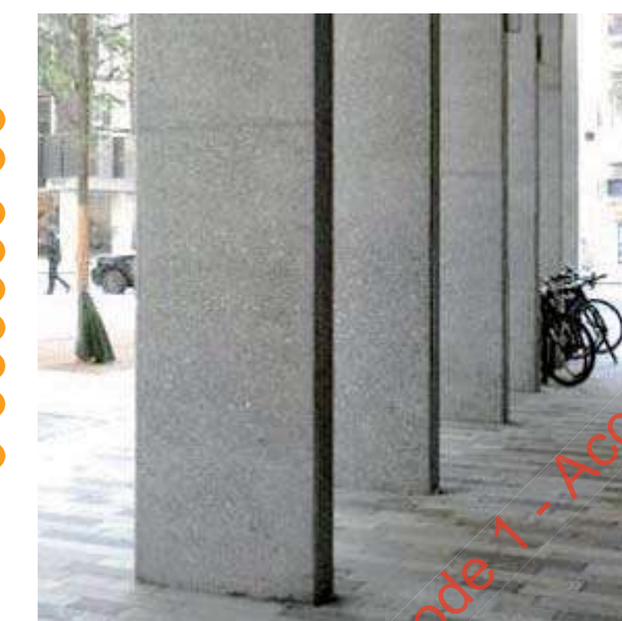
Fig.5.42 Examples of pre-cast concrete colonnade
