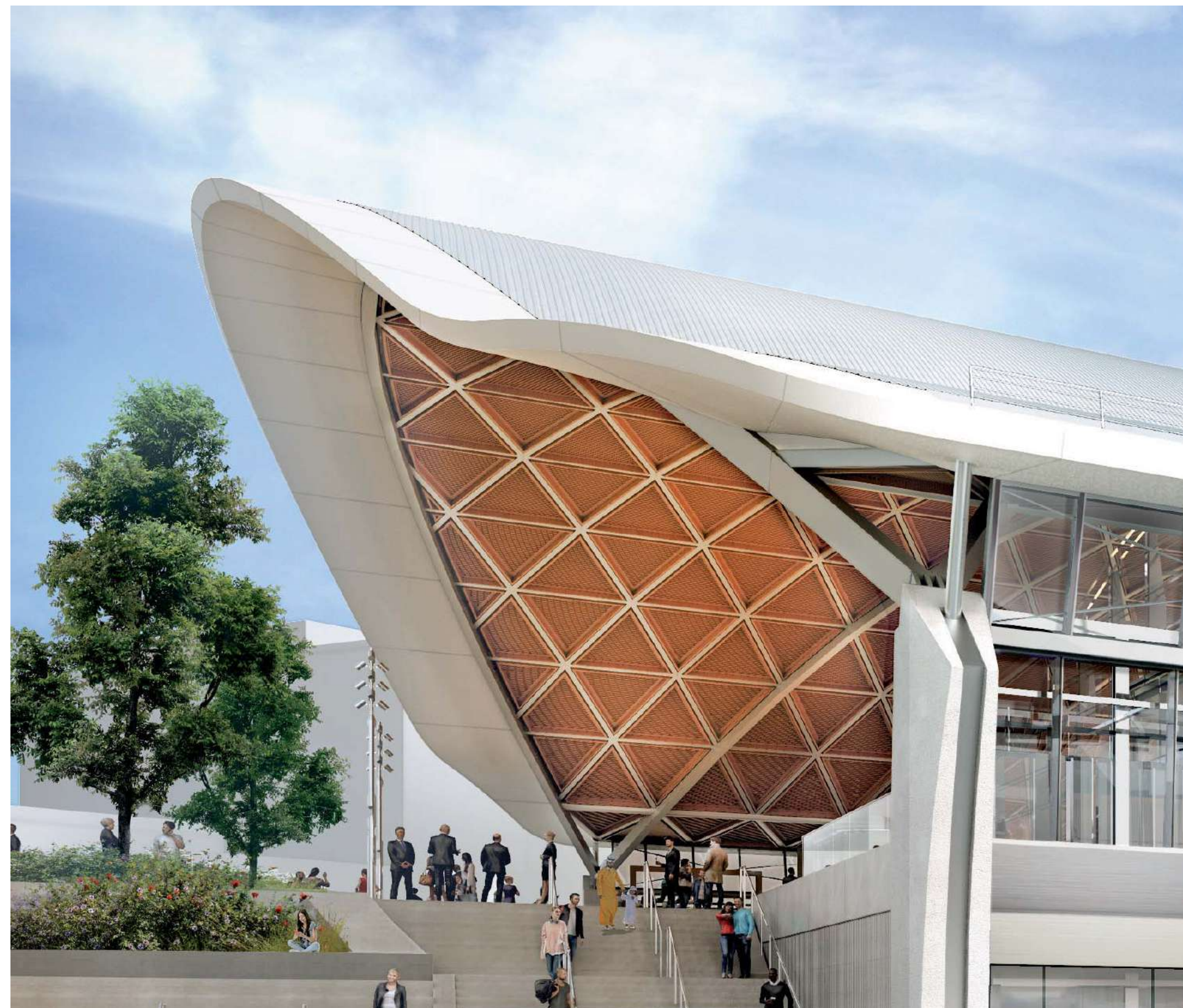
Fig.5.11 Perimeter fascia - Illustration of double curved corner
