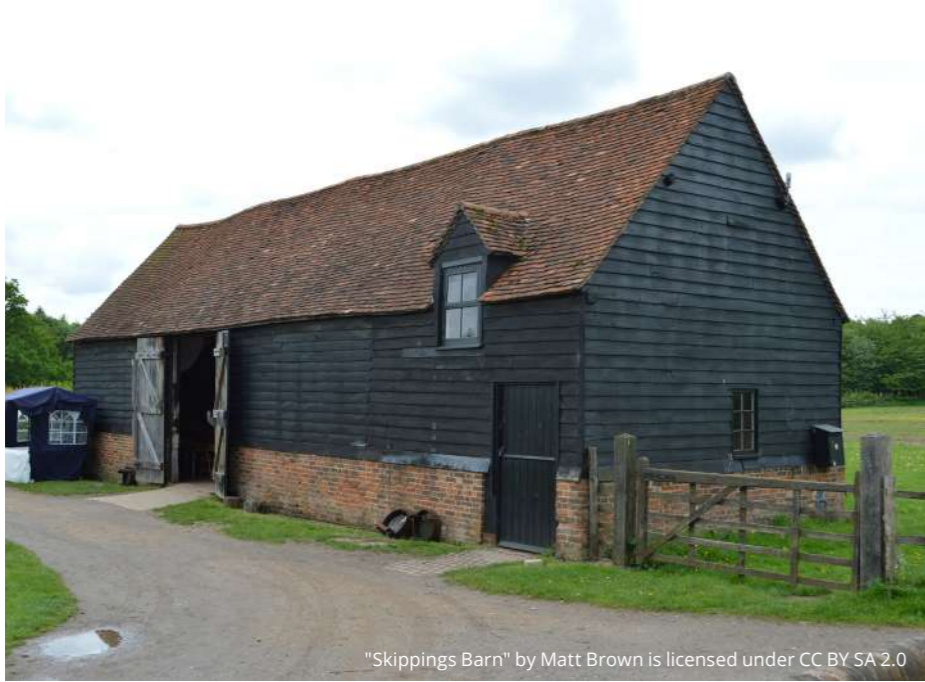
A Fig.2.18_ Photograph - Skippings barn
