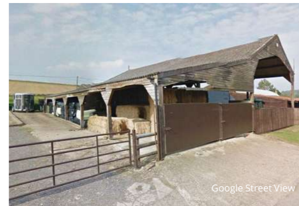
Fig.5.17_ Photograph - Lower bottom house barn
