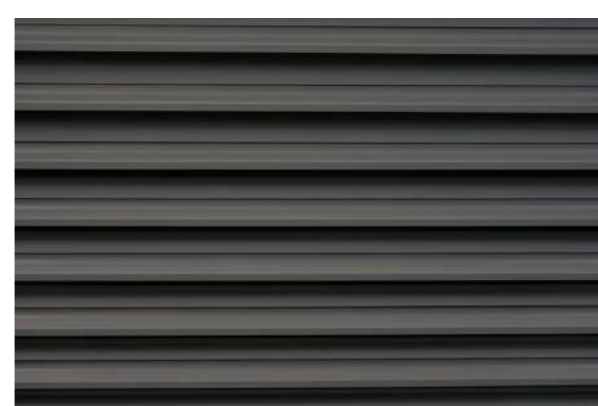
Fig.5.20_ Louvred gable - Painted steel
