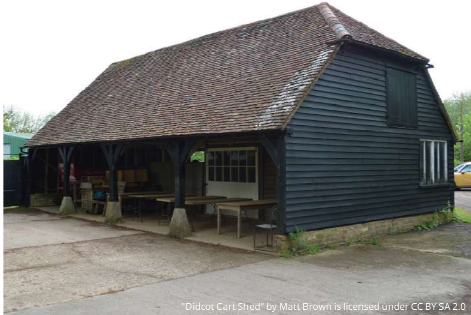
B Fig.2.20_ Photograph - Didcot cart shed
