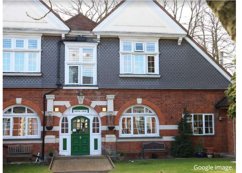
C Fig.2.13_ Photograph - Greene House, Chalfont St Peter
