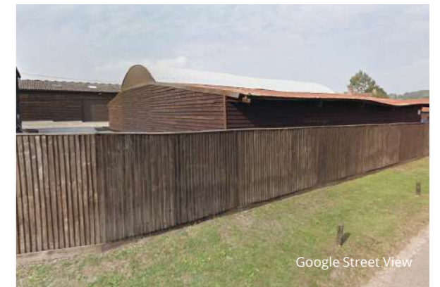
Fig.5.18_ Photograph - Lower bottom house barn
