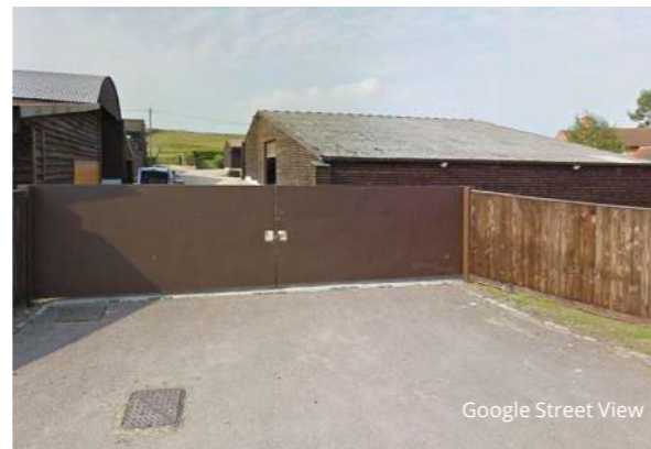
Fig.5.16_ Photograph - Lower bottom house barn
