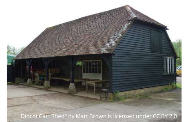
Fig.5.15_ Photograph - Didcot cart shed
