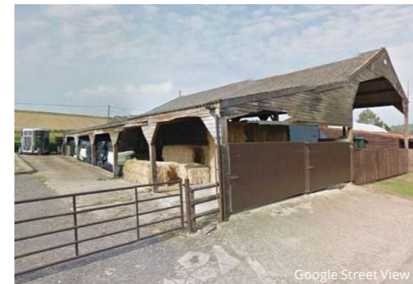
Fig.5.24_ Photograph - Lower bottom house barn
