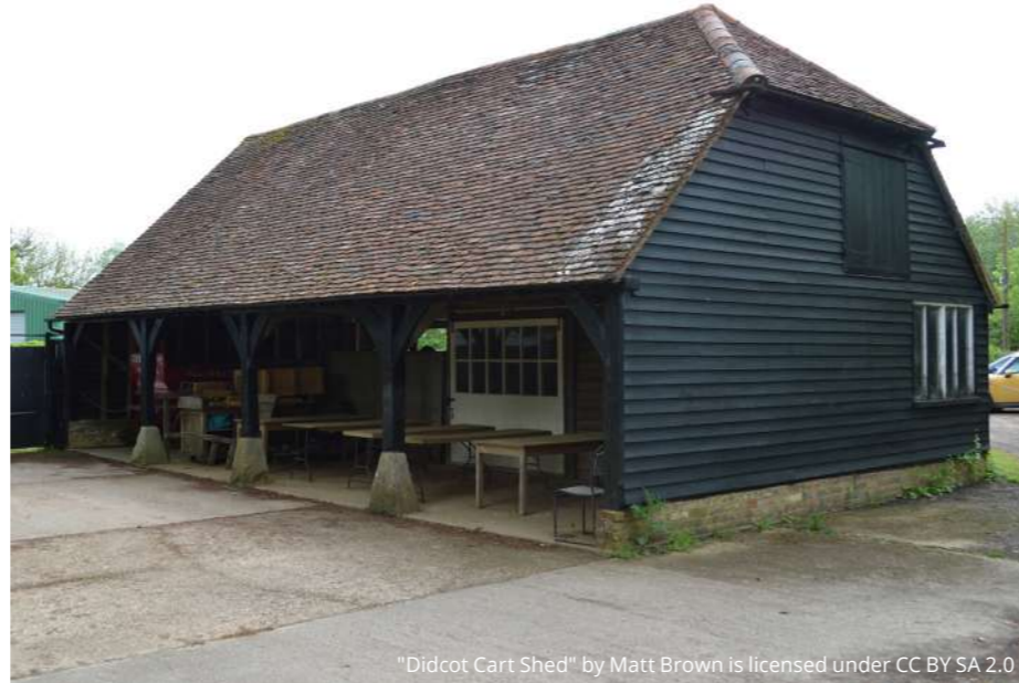
B Fig.2.21_ Photograph - Didcot cart shed
