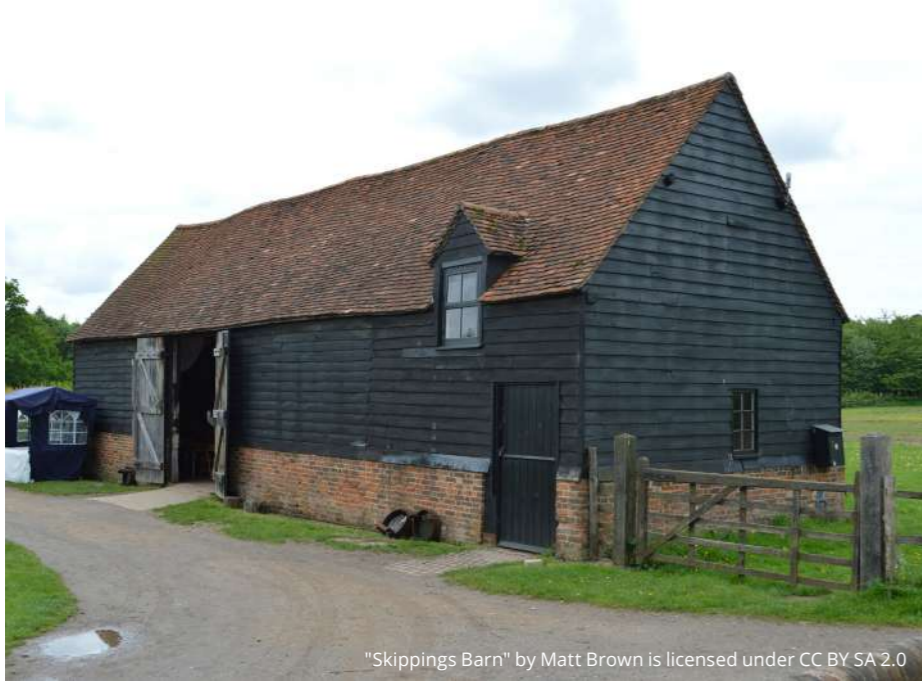
A Fig.2.19_ Photograph - Skippings barn
