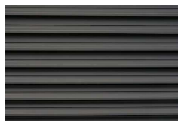
Fig.5.27_ Louvred gable - Painted Steel
