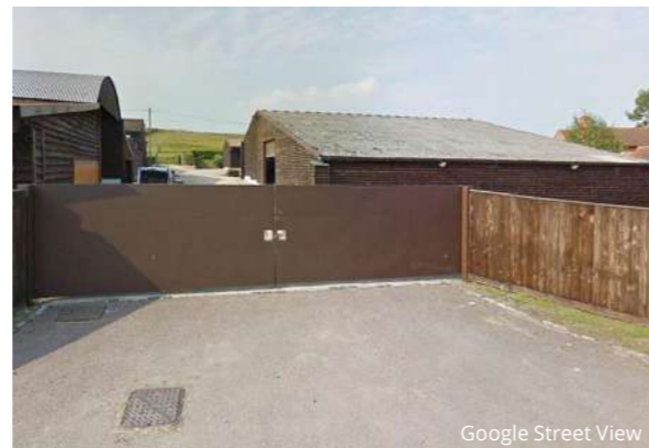
Fig.5.23_ Photograph - Lower bottom house barn
