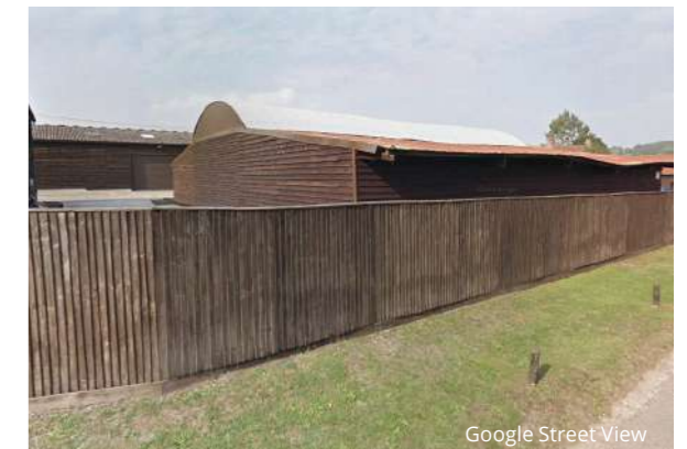
Fig.5.25_ Photograph - Lower bottom house barn
