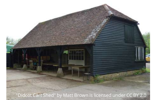
Fig.5.22_ Photograph - Didcot cart shed
