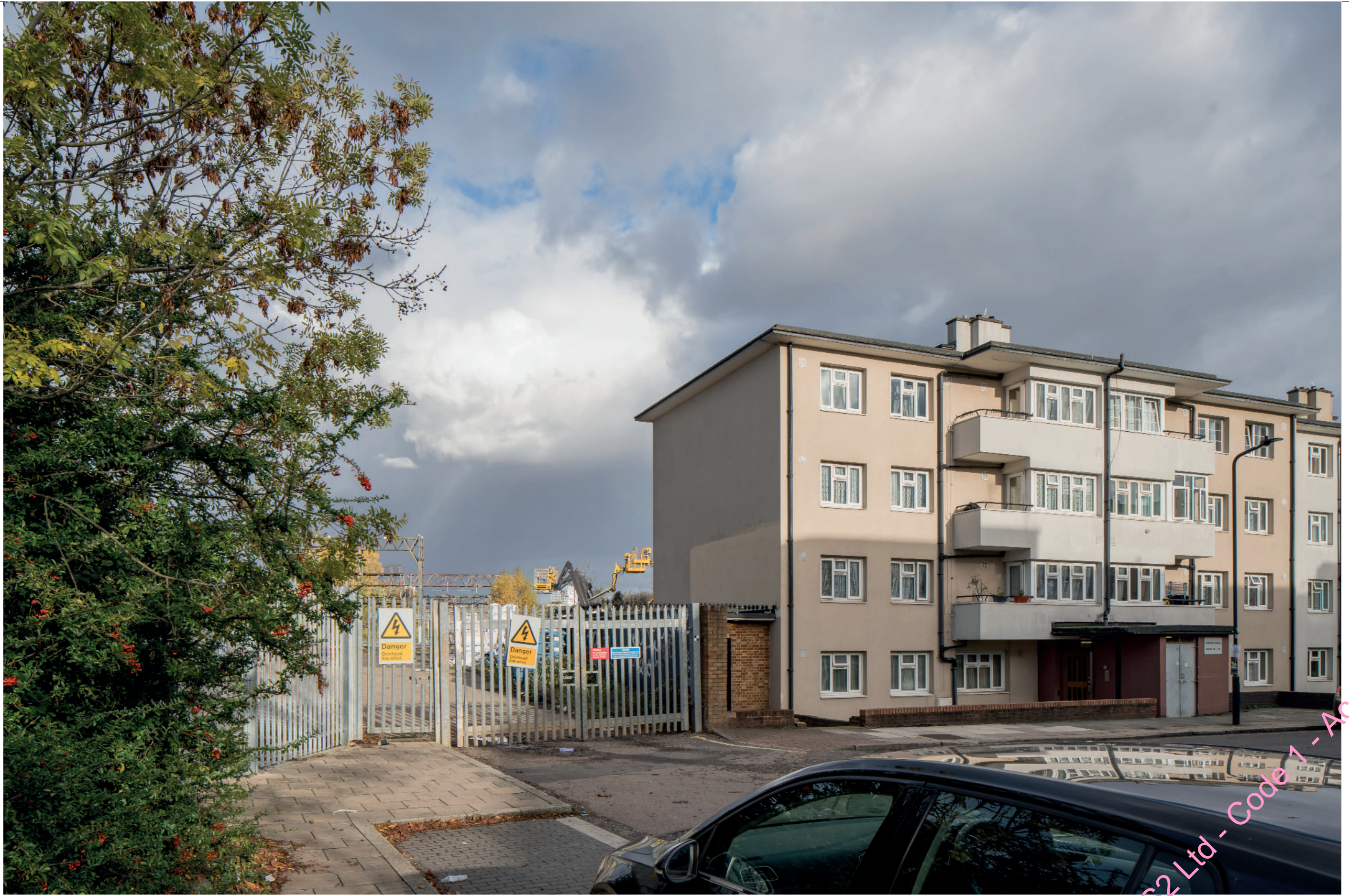
Figure 26: Baseline view of the site entrance on Canterbury Terrace
