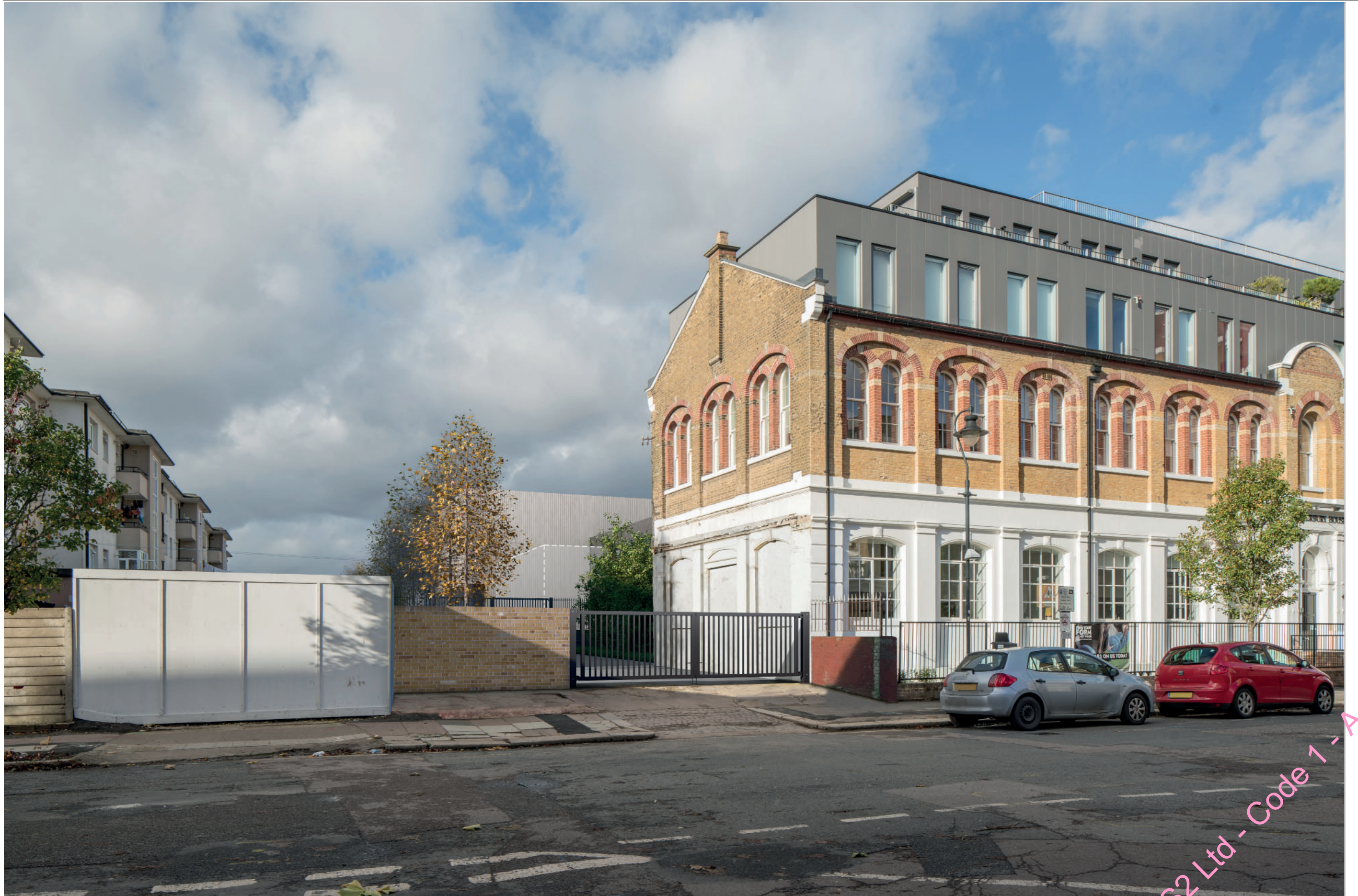
Figure 25: View of the site entrance on Canterbury Road in year 15
