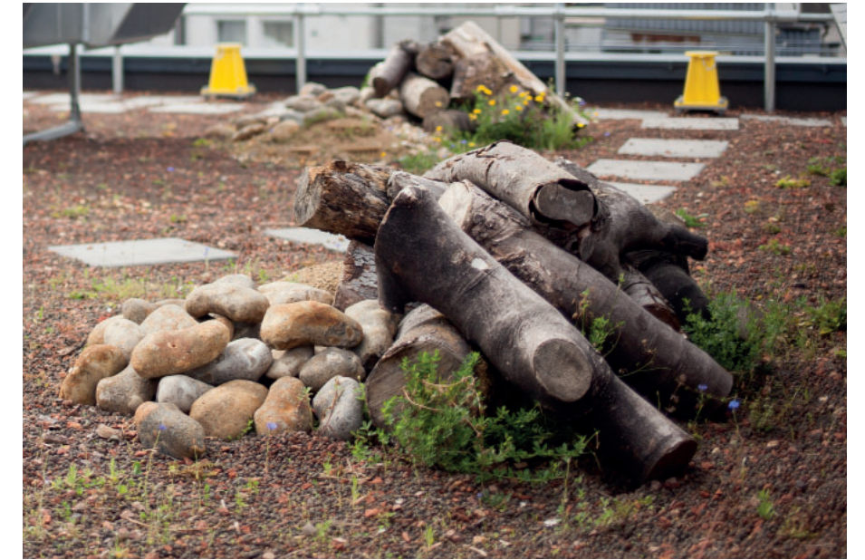
Ecological habitat creation, log piles and rock piles on biodiverse green roof
