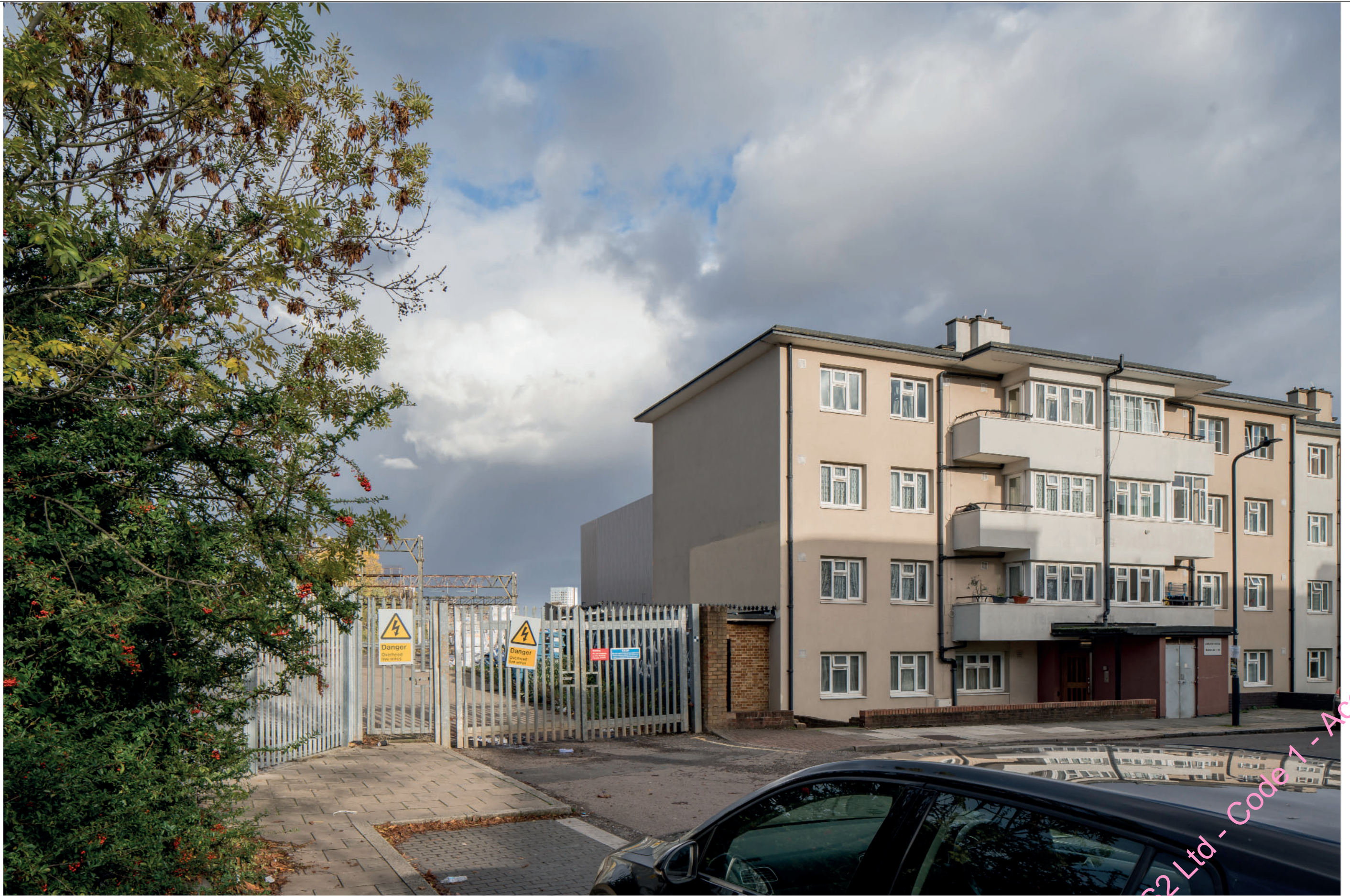
Figure 27: View of the site entrance on Canterbury Terrace in year 1
