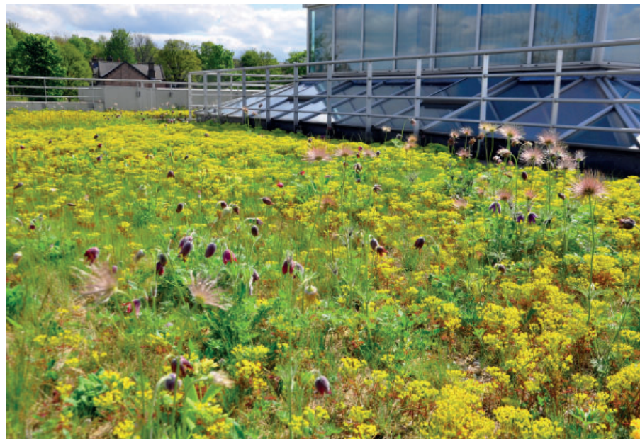
Creation of low maintenance habitats on deep substrate green roof
