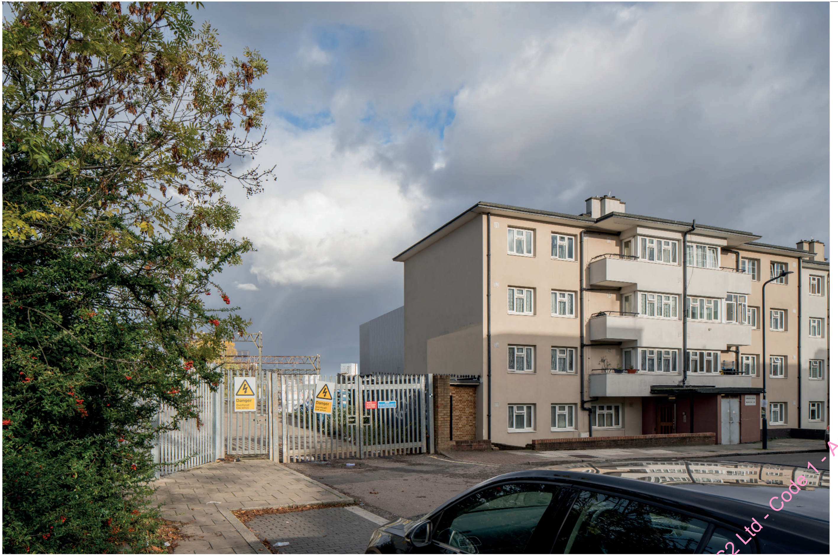
Figure 28: View of the site entrance on Canterbury Terrace in year 15
