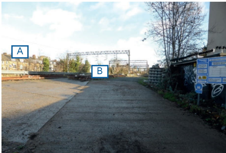
View of Network Rail tracks to the north of the site. Residential dwellings on Brondesbury Villas are located at point A and Network Rail tracks are located at B.
