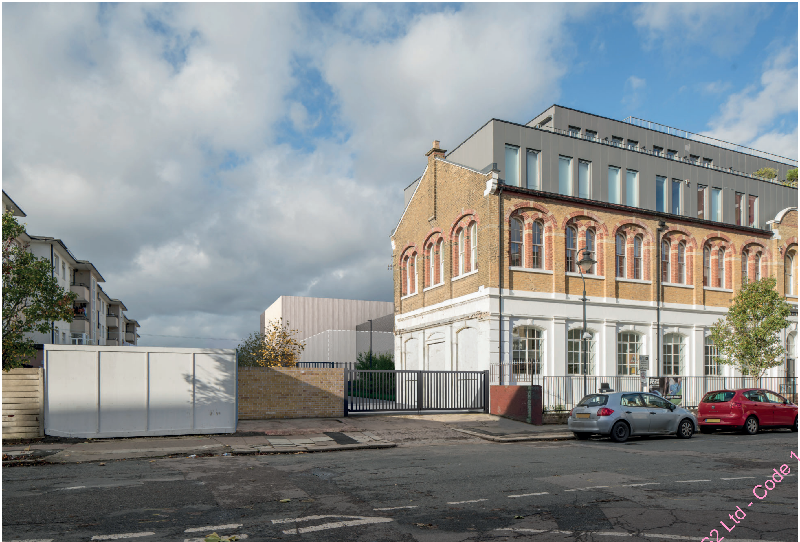
Figure 24: View of the site entrance on Canterbury Road in year 1
