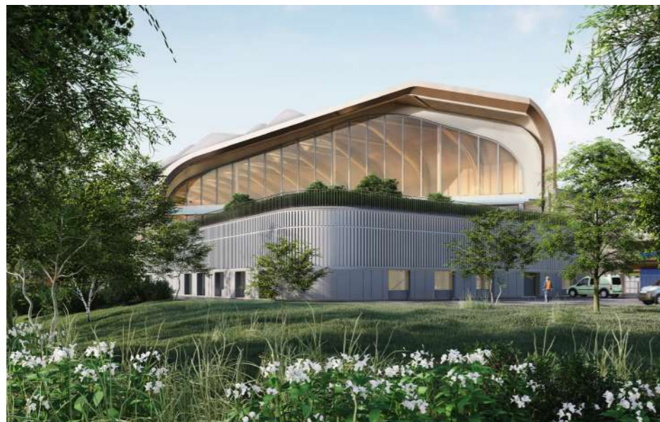
Figure 75: Artist's impression of south end of the building showing rainscreen cladding with integrated doors, windows and air intake/exhausts concealed behind
