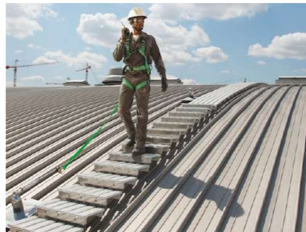
Figure 127: Indicative walkway and steps over gutters
