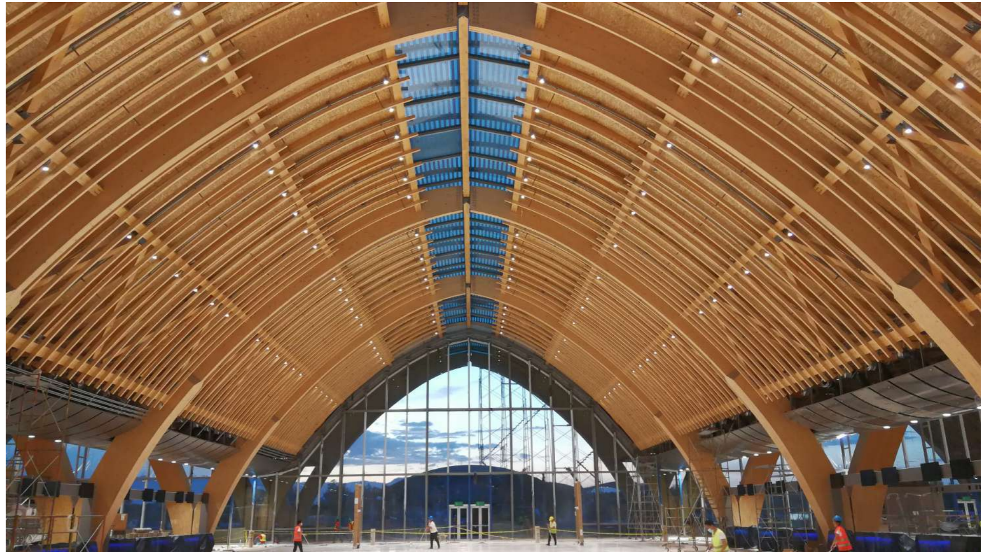
Figure 28: Mactan - Cebu International Airport Terminal 2, Integrated Design Associates with Arup (2018)
