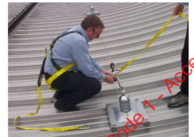
Figure 129: Indicative cableline restraint system
