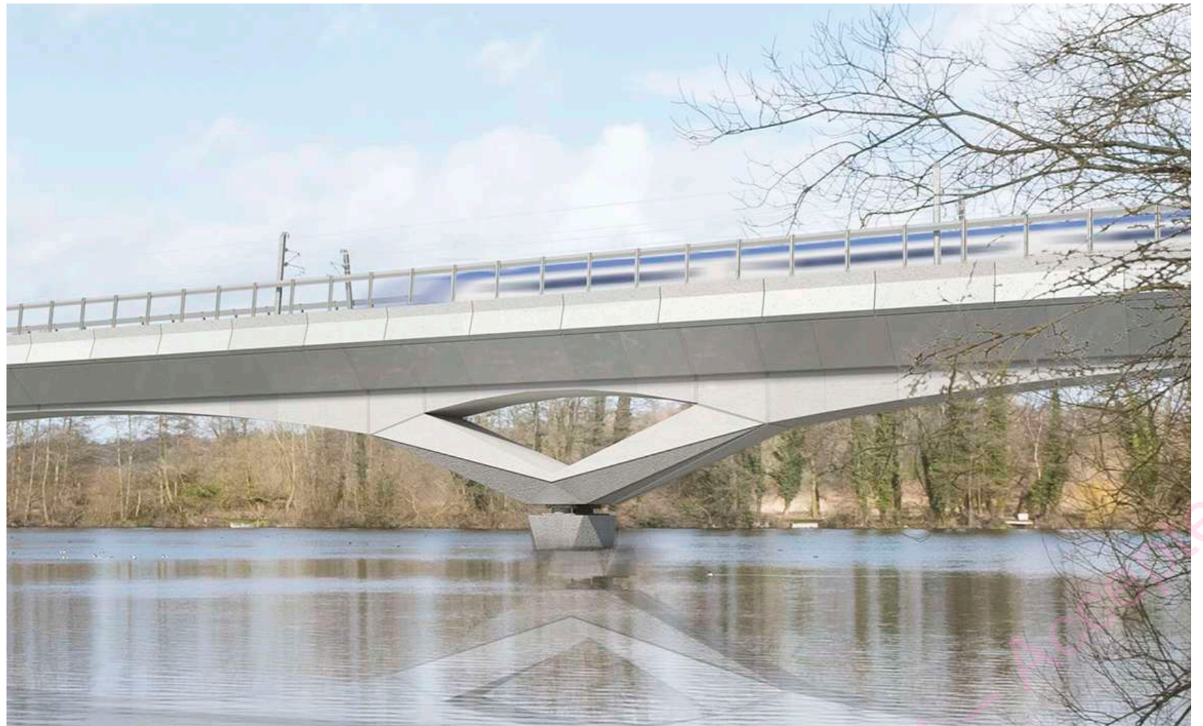
Fig.5.97_ Visualisation (8) - 4m hybrid barrier over Korda Lake
