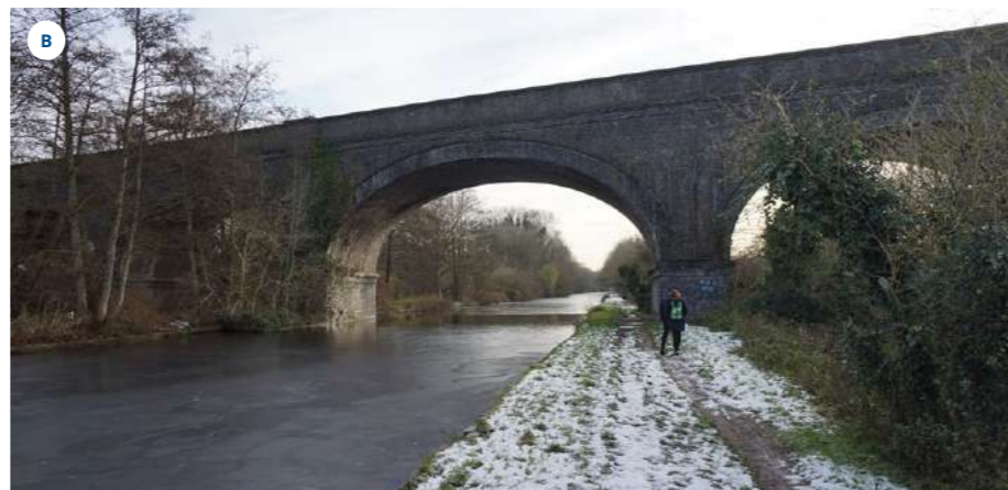
B Fig.2.34_ Photograph - Existing railway crossing Grand Union Canal
