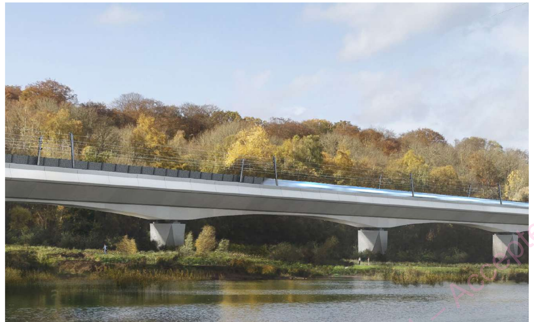
Fig.5.94_ Visualisation (5) - 1.65m opaque barrier along Denham Waterski Lake
