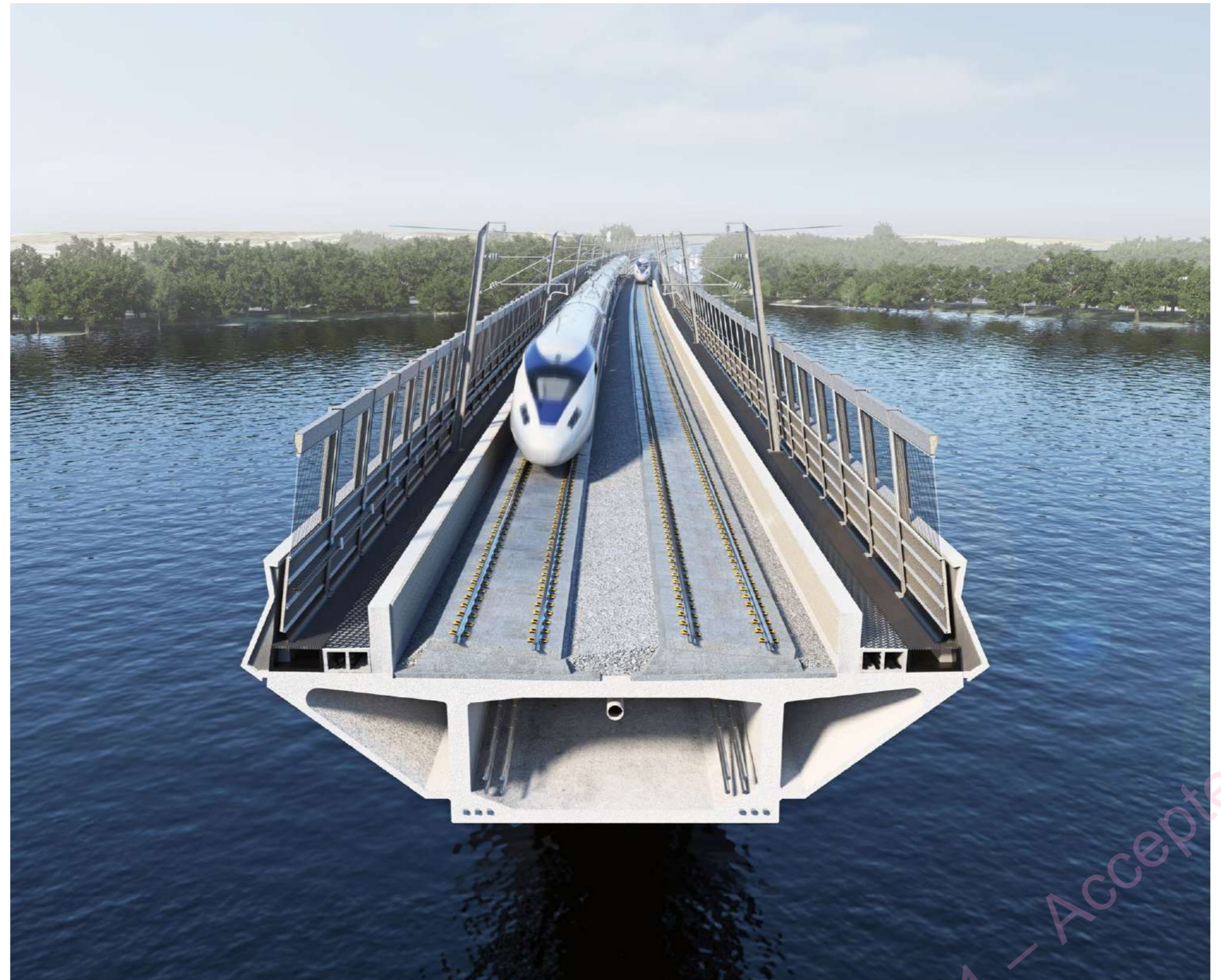
Fig.5.17_ Visualisation (16) - Perspective deck cross section over Harefield No.2 Lake
