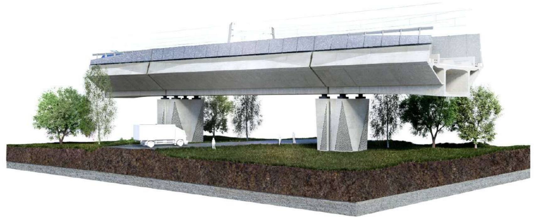
Fig.5.66_ Illustrative view - Expansion portal over Moorhall Road
