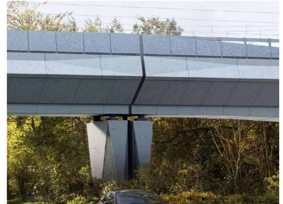
Fig.5.87_ Visualisation - Expansion joint at expansion portal
