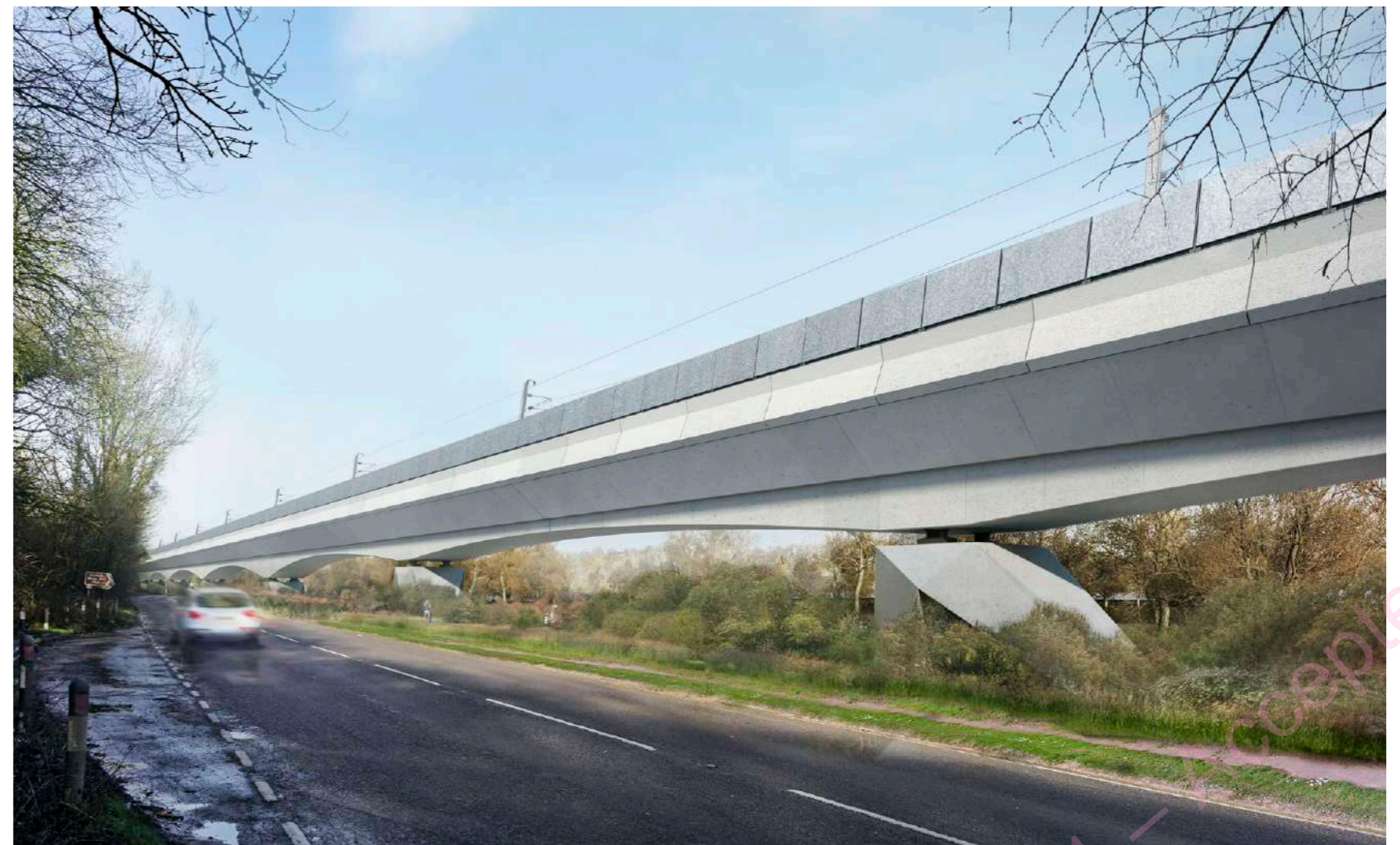
Fig.5.100_ Visualisation - 4m opaque barrier along the A412
