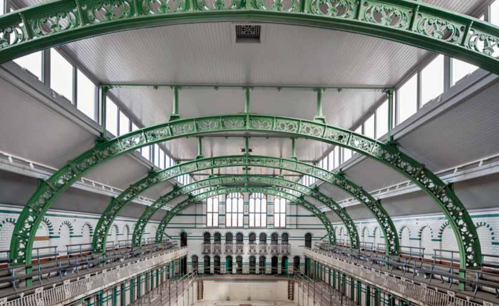
Restored Cast Iron Trusses, Moseley Road Baths, Birmingham, West Midlands
