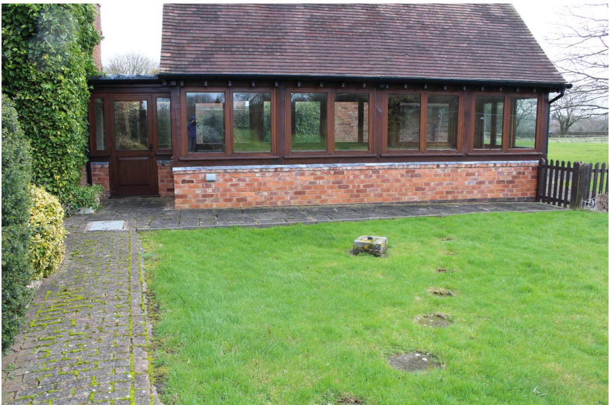
Image EDP 6 View of the area to the south of the main house where the HER suggested foundations of a former building was present. No evidenced of these foundations were observed during the site visit.
