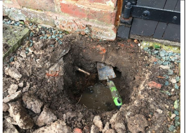
Plate 26 – The foundation of the stable block/outbuildings' S elevation.
