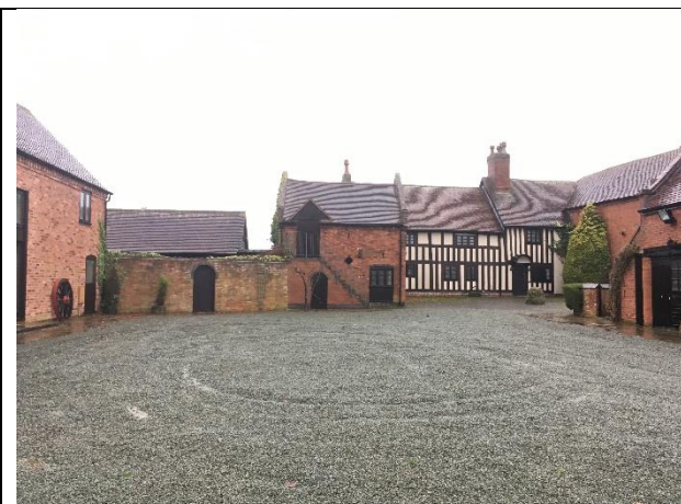
Plate 17 – The central courtyard at Jerrings Hall Farm, looking NW.
