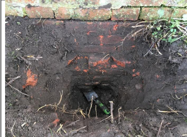
Plate 25 – The foundation of the stable block/outbuildings' N elevation.
