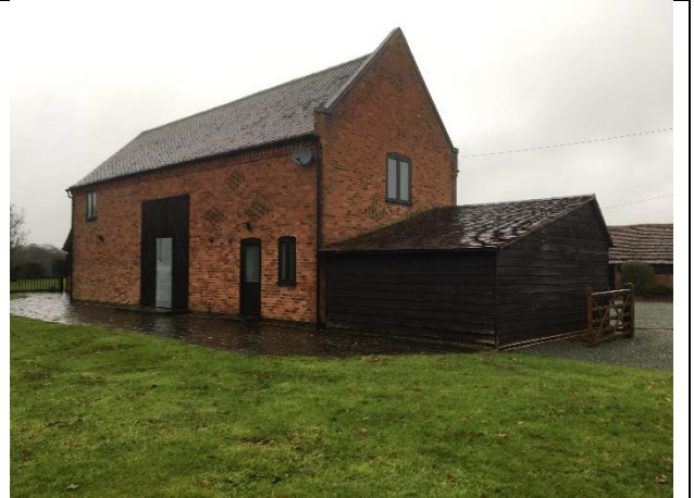
Plate 14 – The S elevation of the barn conversion, looking NW.
