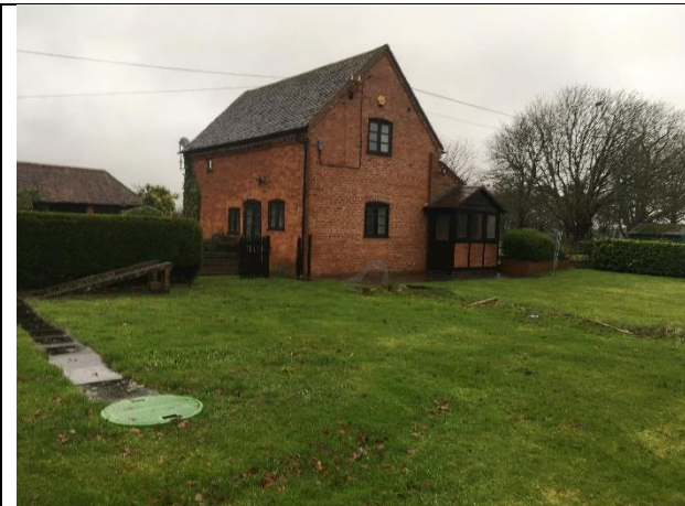
Plate 15 – The S & W elevations of the cottage, looking NE.
