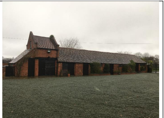
Plate 16 – The S elevation of the stable block/outbuildings, looking NE.
