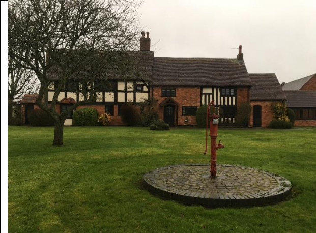
Plate 13 – The W elevation of Jerrings Hall, looking E.
