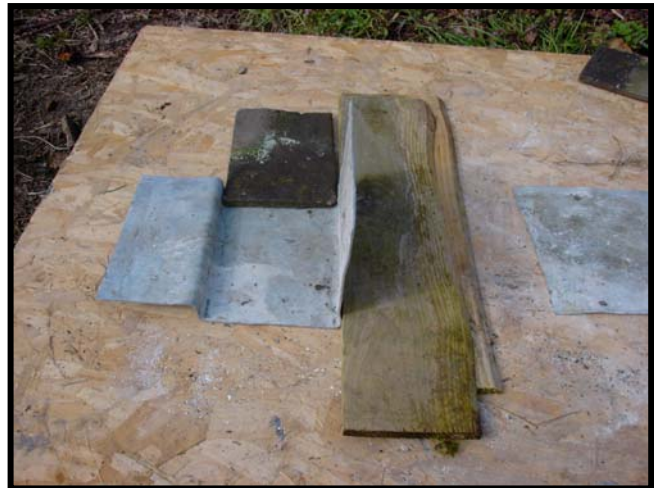
Forming the second 'wing' of the Batslate and the width by using one of the tiles.
