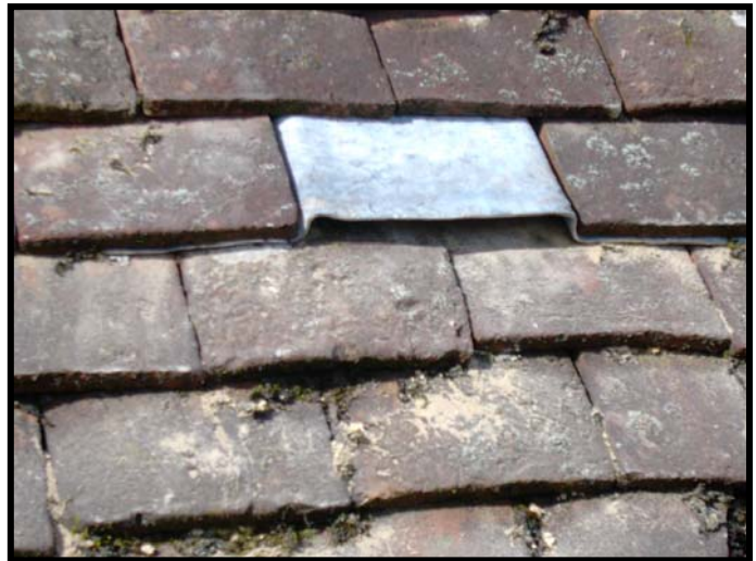
The Batslate with all the surrounding tiles replaced.
