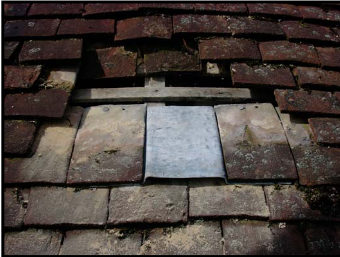
Tiles are refitted around the Batslate.
