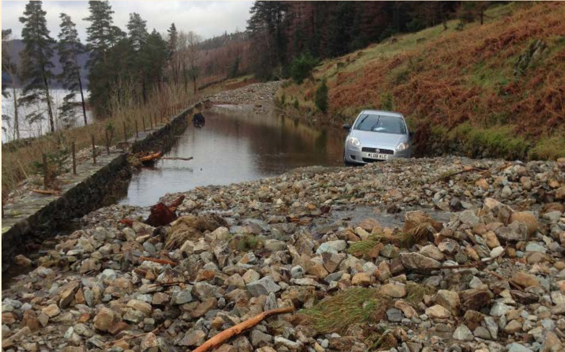
Image: Landslide deposits block the A591 beside Thirlmere (Cumbria County Council©)
