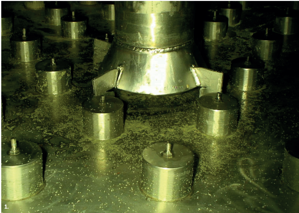
1. High-definition image of ion exchange vessel
