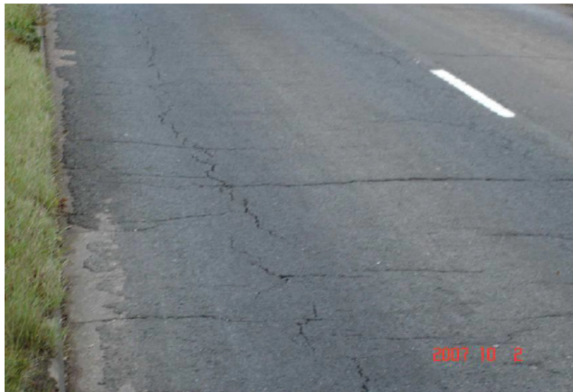
Figure 4: Cracking
