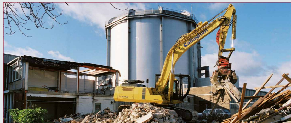
Demolition work at Harwell
