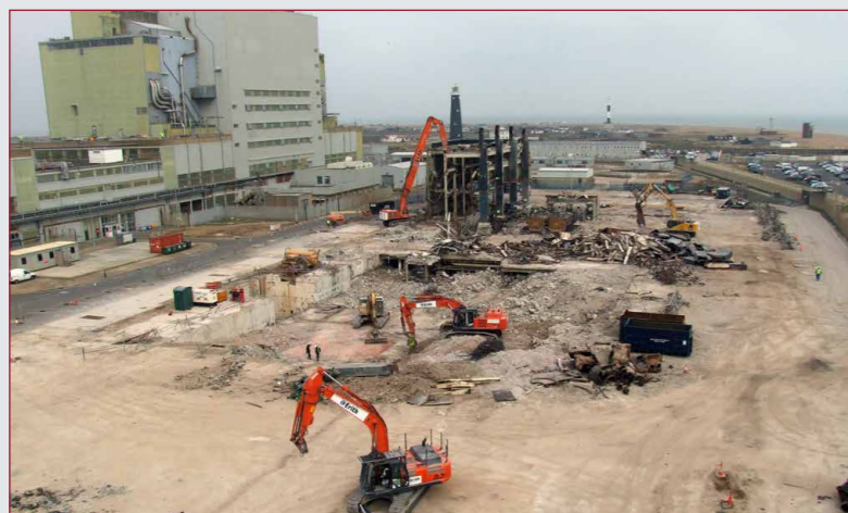
Demolition work at Dungeness
