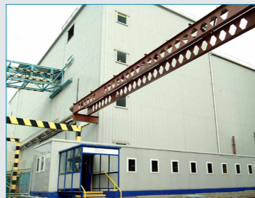
Magnox Reprocessing Plant - Sellafield
