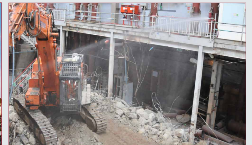
Turbine hall demolitions
