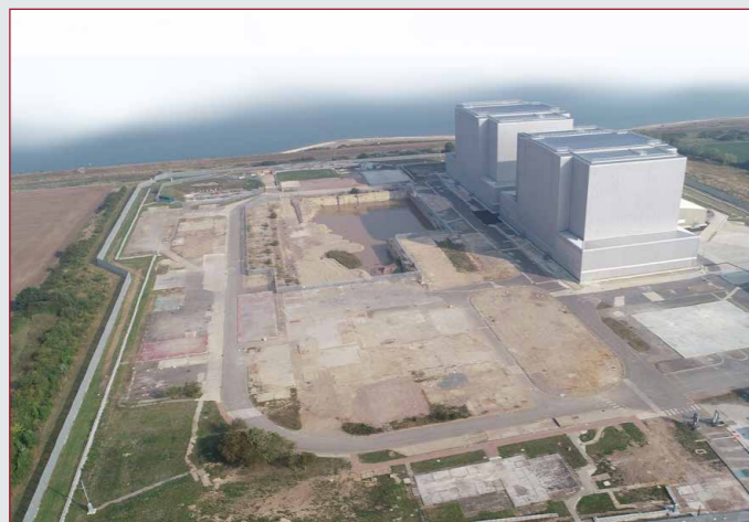
Bradwell in care and maintenance
