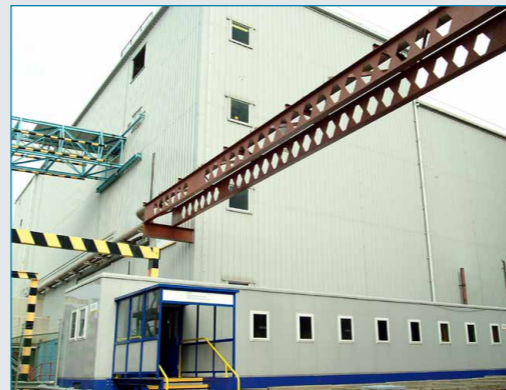
Magnox Reprocessing Plant - Sellafield
