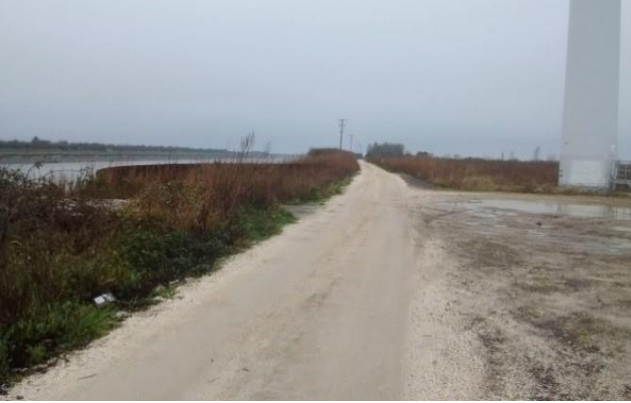
Top: BOAT running alongside the river. Also shows a loop (grey surface) that has been put in so the turbine blades do not oversail the BOAT.
