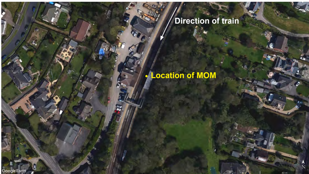
Figure 2: Aerial view of Rowlands Castle station showing the direction of travel of the train and the approximate location of the MOM immediately before the incident
