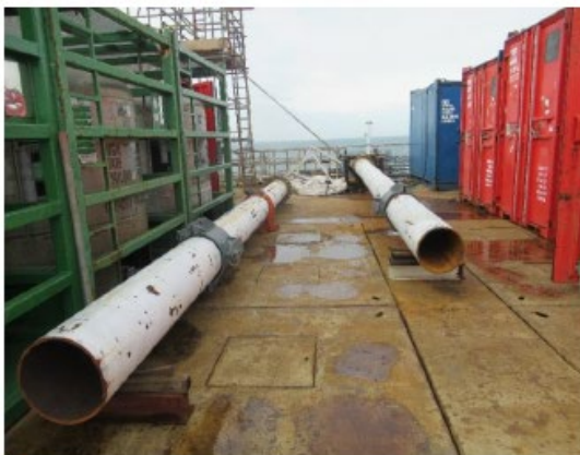
Figure 1 - Vent Stack during removal, lifting, laydown and post-removal
