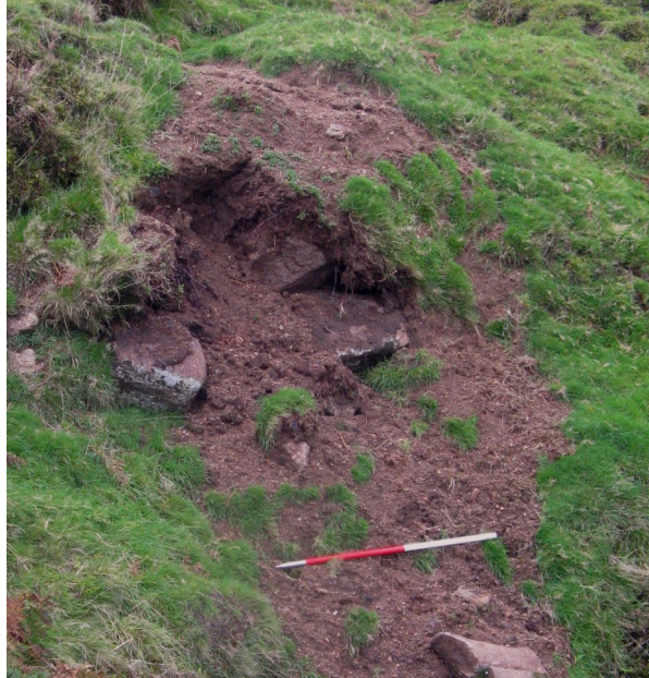
Fig 12 1300628, 2013. Burrowing animal damage at Eylesbarrow Mine
