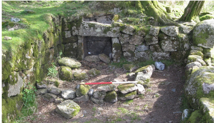
Fig 4 Detail of recently constructed shelter in the ruined building 441725.
