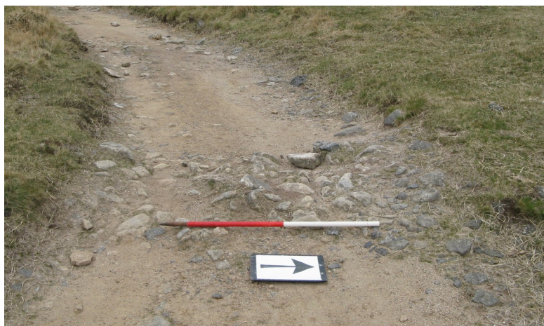
Fig 5 1450575. Reave at threat from foot and cycle damage
