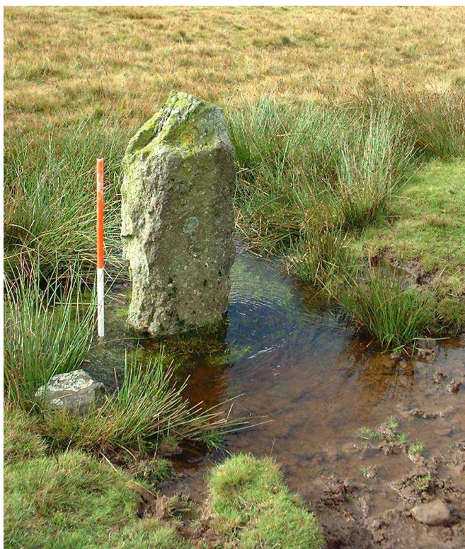
Fig. 6 Boundary stone 1403757. Despite the large water-filled hollow at the foot of this stone it remains secure in its socket.
