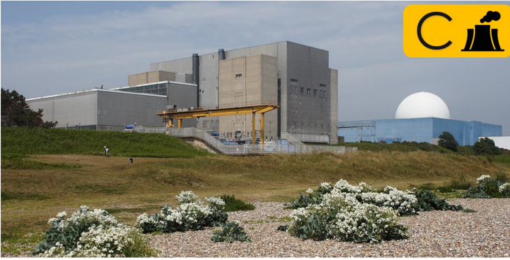
Sizewell A (1966-2006) and B (1995-) Nuclear Power Stations (6/13 lu05) by Ted and Jan is licensed under CC BY 2.0
