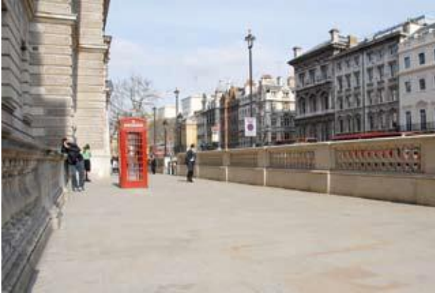
Figure 2.3 Structural balustrades in Whitehall, London
