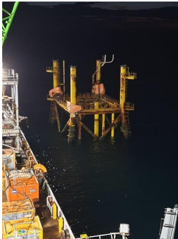
Figure 9.5.2: Markham ST-1 Jacket without topsides
