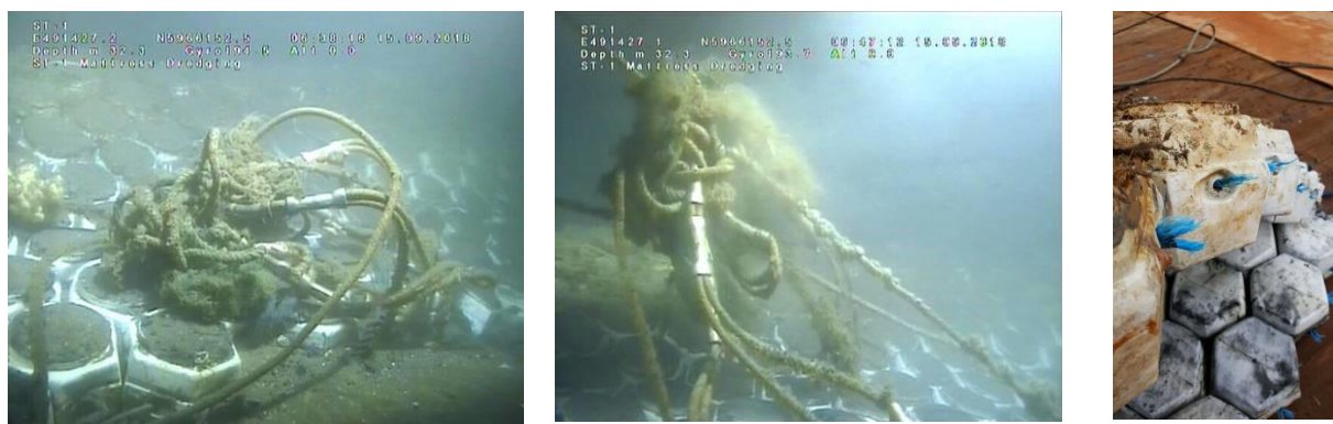
Figure 4.2.3: Concrete mattresses & rigging, failed polypropylene rope
