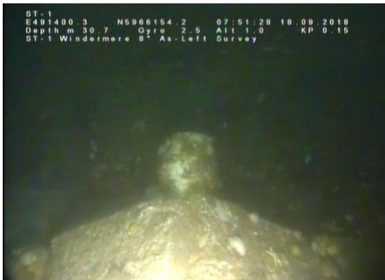
Figure 4.2.5: Windermere pipeline PL1273 severed (mattress in foreground)
