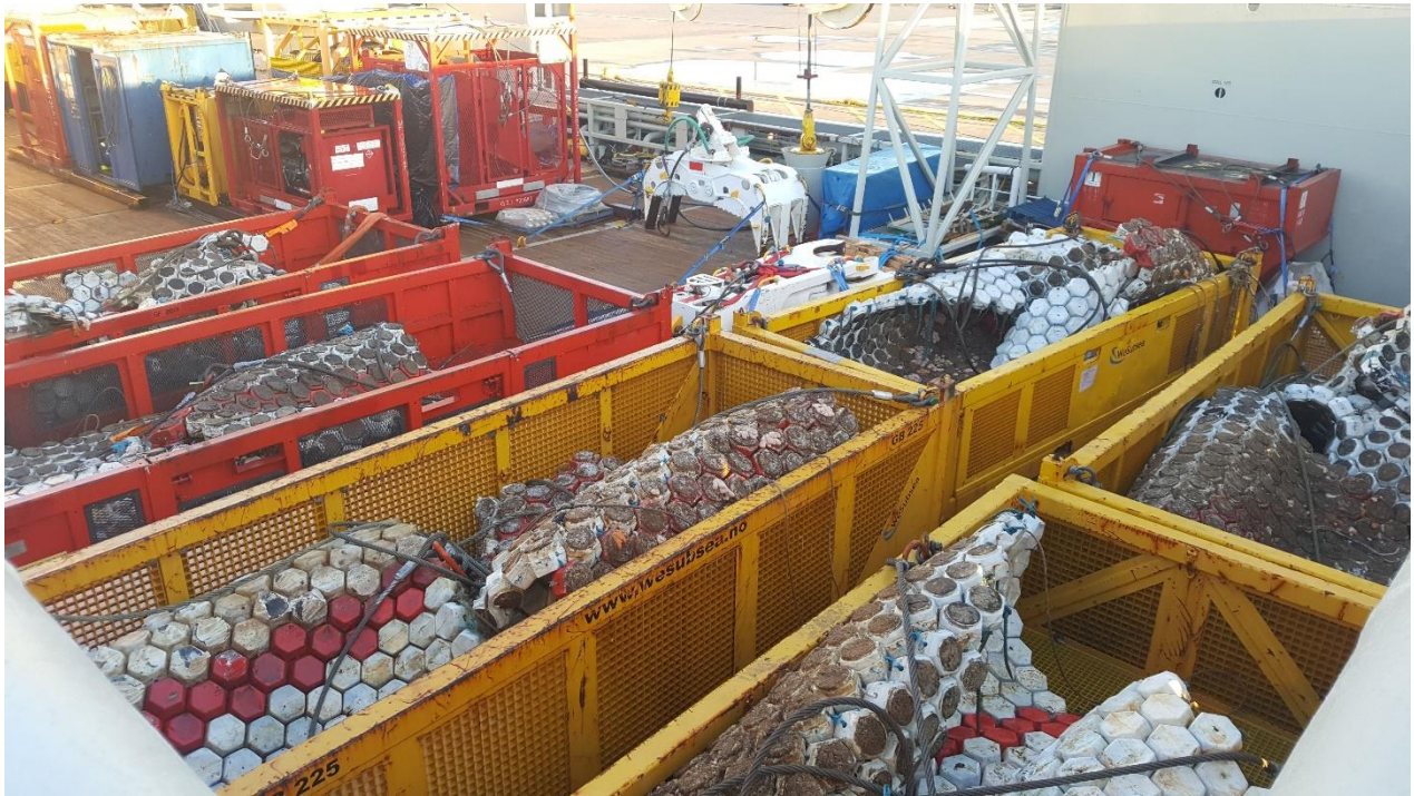
Figure 9.2.1: Concrete mattresses recovered in baskets
