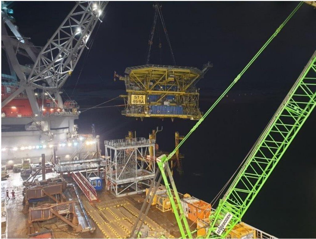
Figure 9.5.1: Markham ST-1 Topsides about to be lifted
