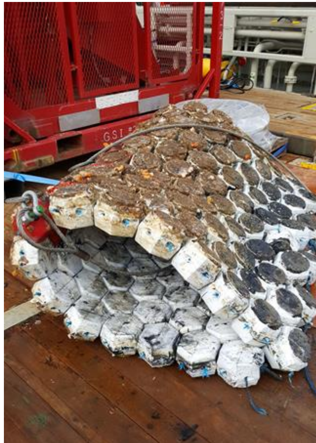
Figure 9.2.2: Loose concrete mattress
