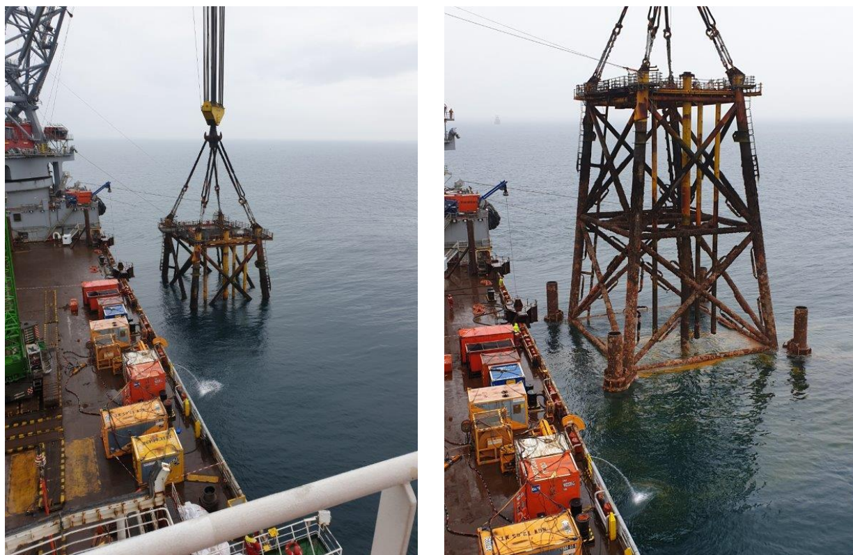
Figure 9.5.3: Markham ST-1 Jacket being recovered
