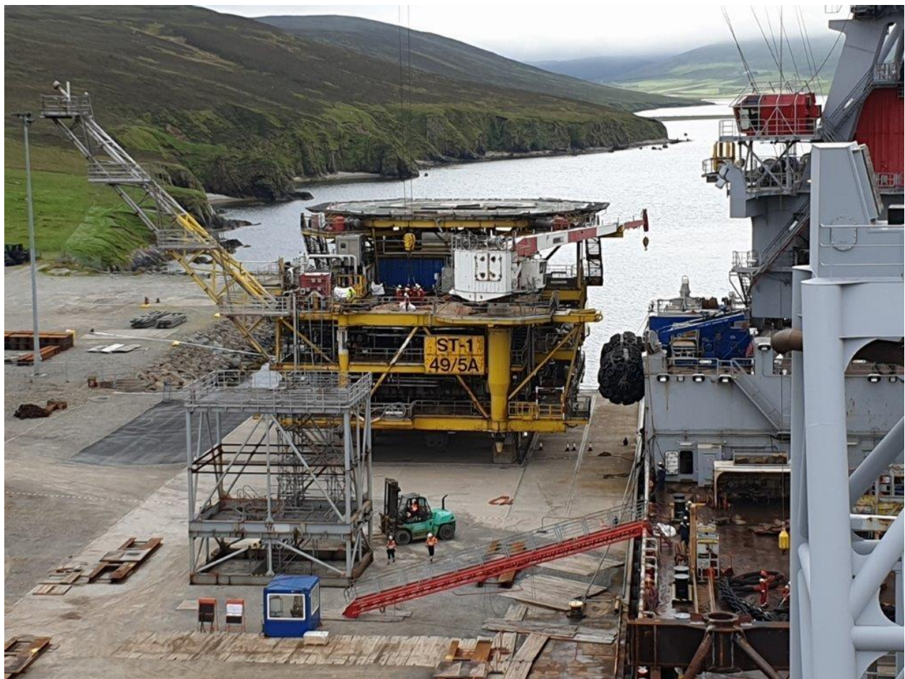
Figure 9.8.2: Markham ST-1 Topsides fully landed
