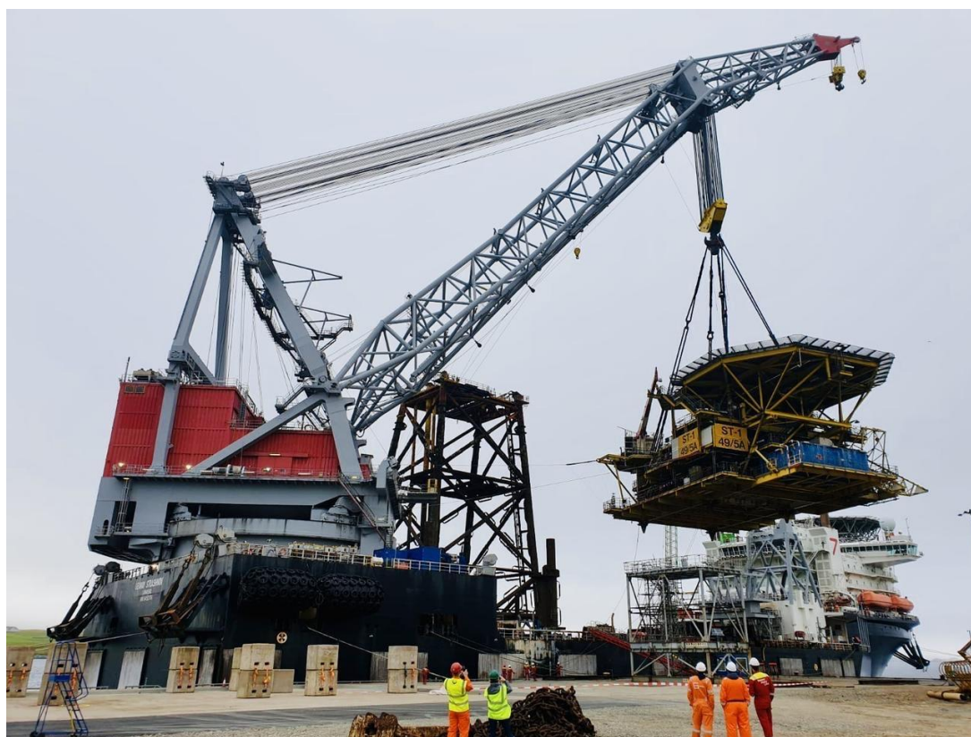
Figure 9.7.1: Markham ST-1 Topsides being lifted to shore
