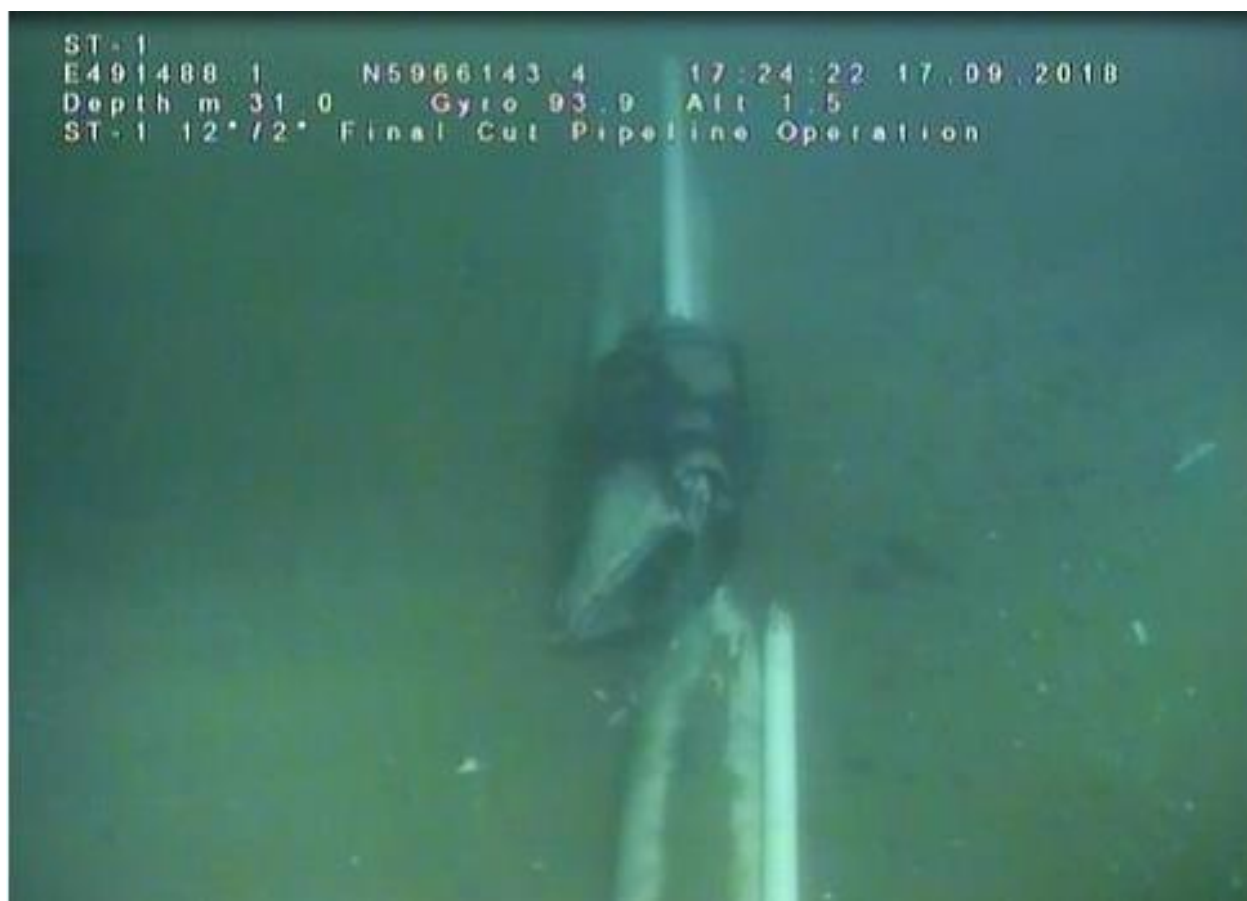
Figure 4.2.4: PL992 & PL993 both severed
