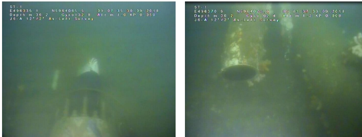
Figure 4.2.6: PL992 & PL993 severed at J6A @mattresses and riser)
