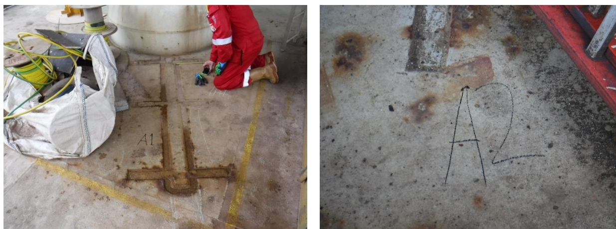
Figure 9.4.1: Reinstating the Topsides Lifting Padeyes (Leg A1 & A2)
