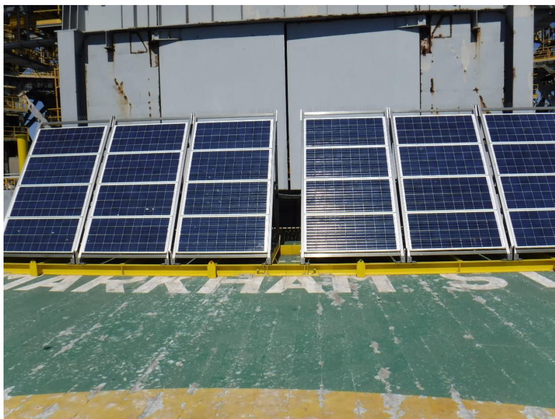
Figure 9.3.2: Solar Panels mounted on Helideck
