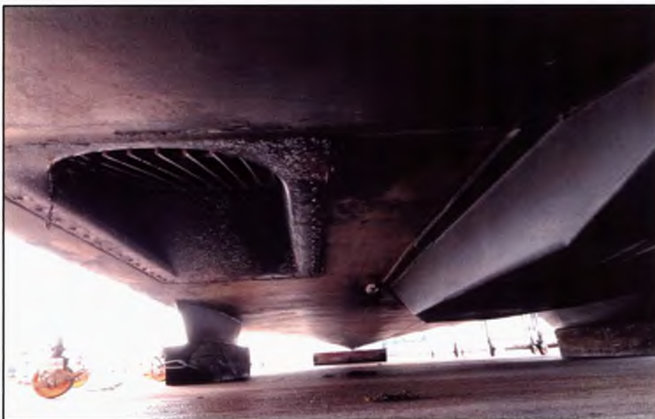
Figure 1.4.21 – LCVP Port Water Inlet Duct viewed from below and rear.
