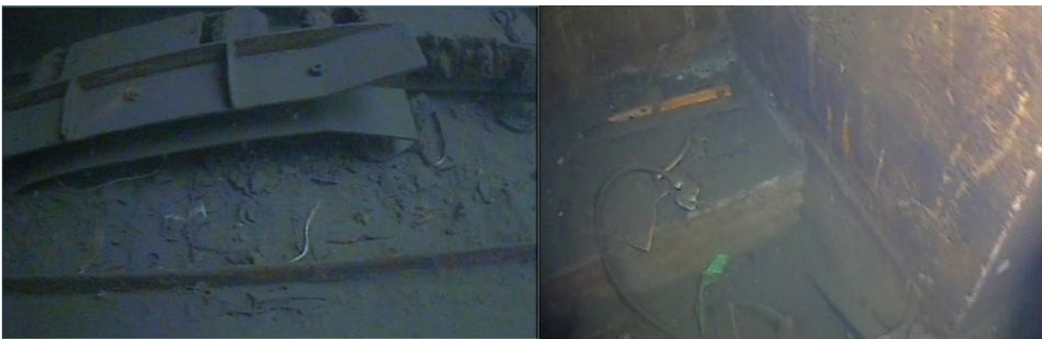
Figure 34: PFSP Bays 11 and 12 showing solid debris and sludge
