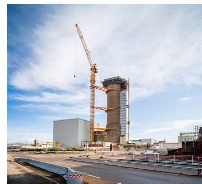
Figure 46: Tower crane on the side of the Windscale chimney pile 1
