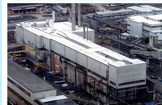
Figure 38: Magnox Swarf Storage Silo
