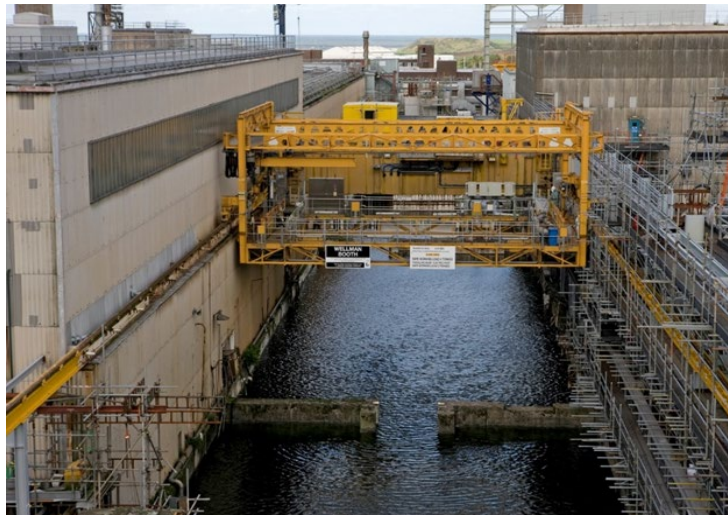
Figure 28: First Generation Magnox Storage Pond
