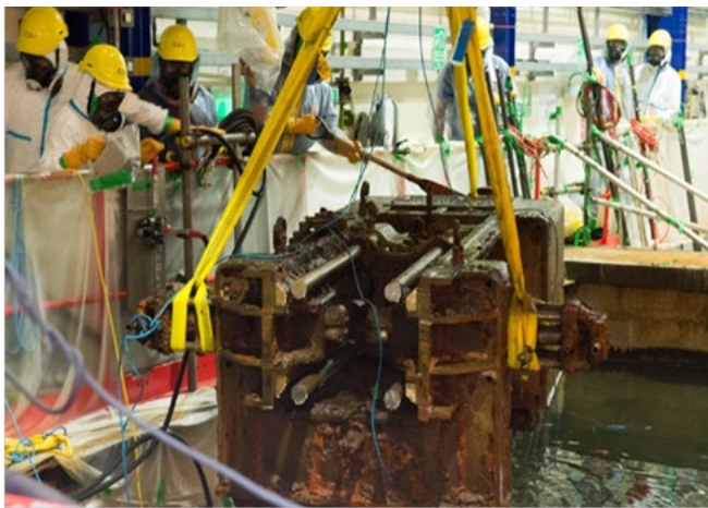
Figure 30: Example of the removal of a bulk solid item from ponds
