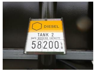
Figure 6 – Typical Tank Sign at Fill Point(s).
