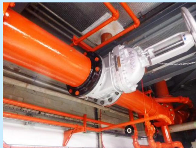
Figure 23 – Completed remediation on gas circulator fire pipework
