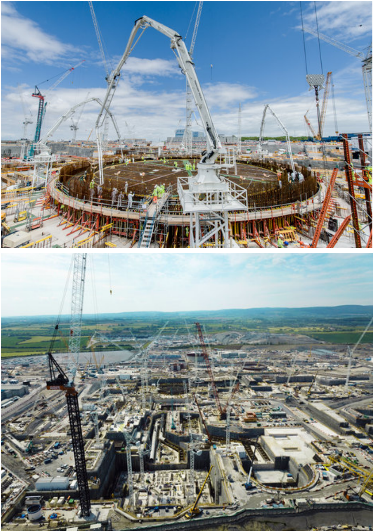
Figure 1 and 2 – Construction at Hinkley Point C
