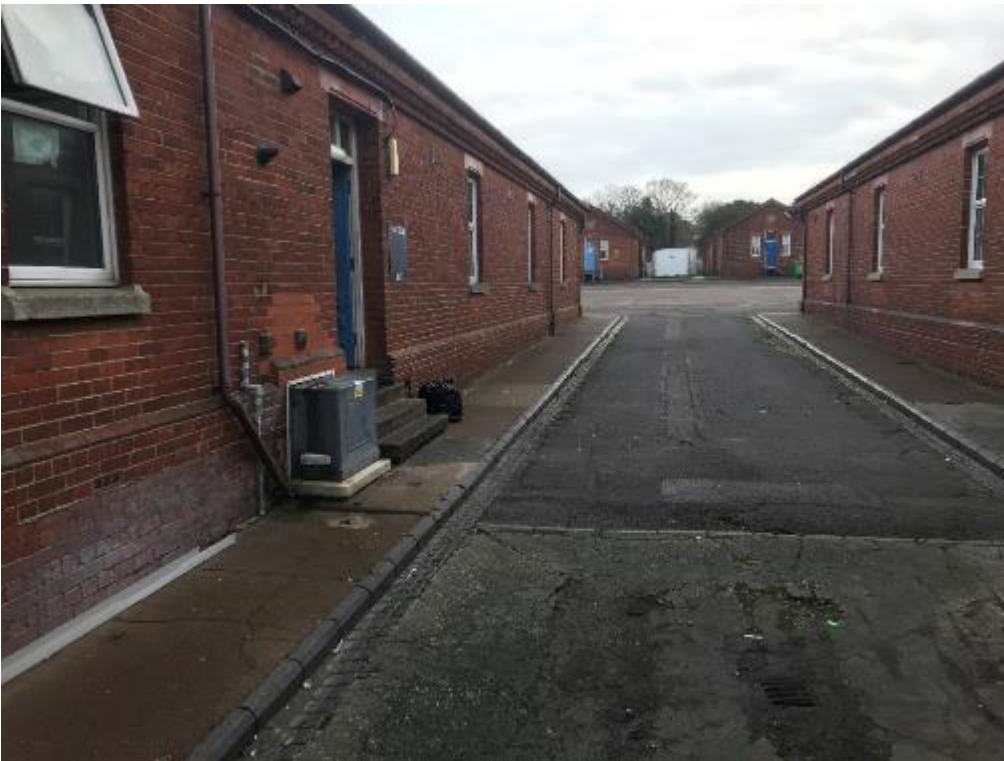
Outside of billets, Napier Barracks
