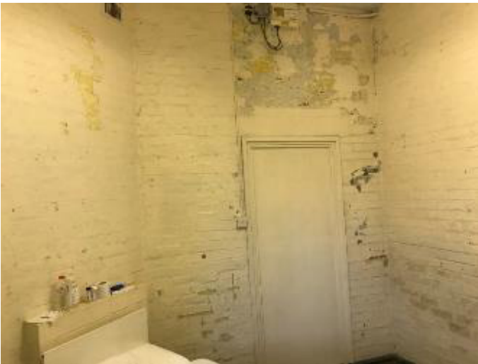
Currently occupied isolation unit room, Napier Barracks
