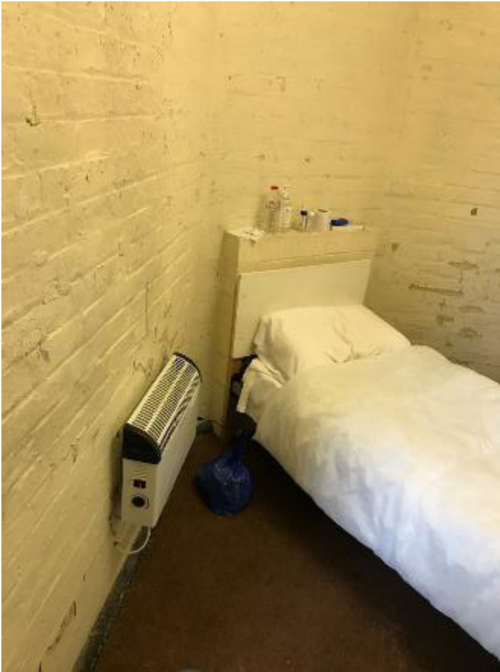
Currently occupied isolation unit room, Napier Barracks
