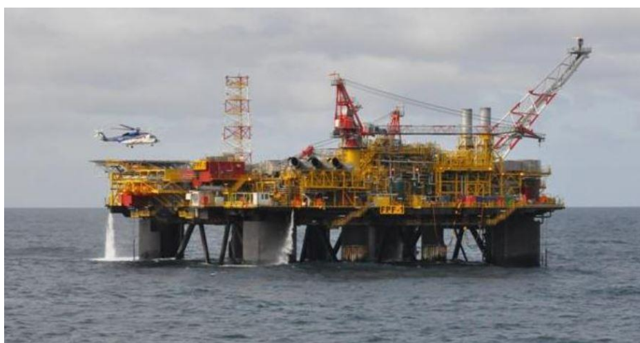
Figure 3.15 – The FPF-1 facility
